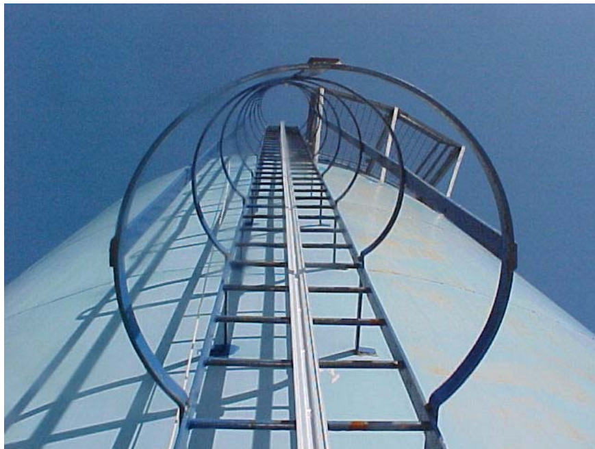
Photo # 4—STGTGS--- Fuel Storage Tank with T-Rail Attached to Ladder
