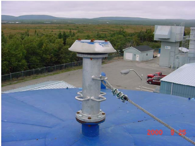
Photo # 5—STGTGS Fuel Storage Tank with Safety Wire Attached to Tank Center Vent
