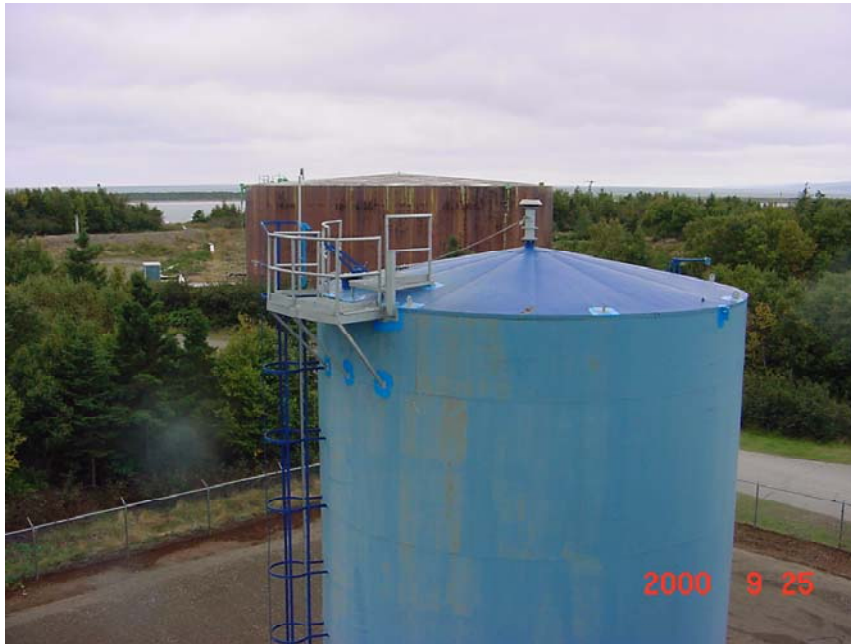
Photo # 3—Stephenville Gas Turbine Generating Station (STGTGS) Fuel Storage Tank with T-Rail Attached to Ladder and Safety Wire Attached to Tank Center Vent
