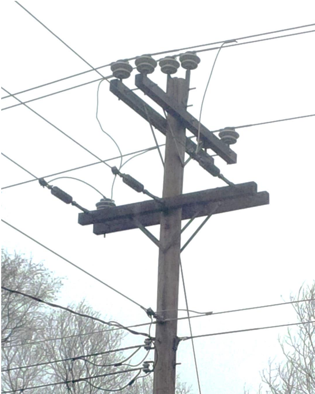
Figure 1 – GFS-02 Main Trunk 2-Piece Insulators
