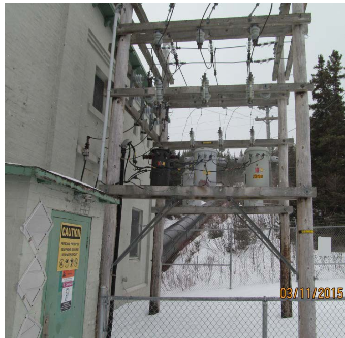
Figure 1 – Low Voltage Substation
