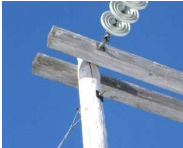
Figure 2: Deteriorated Wood Pole
