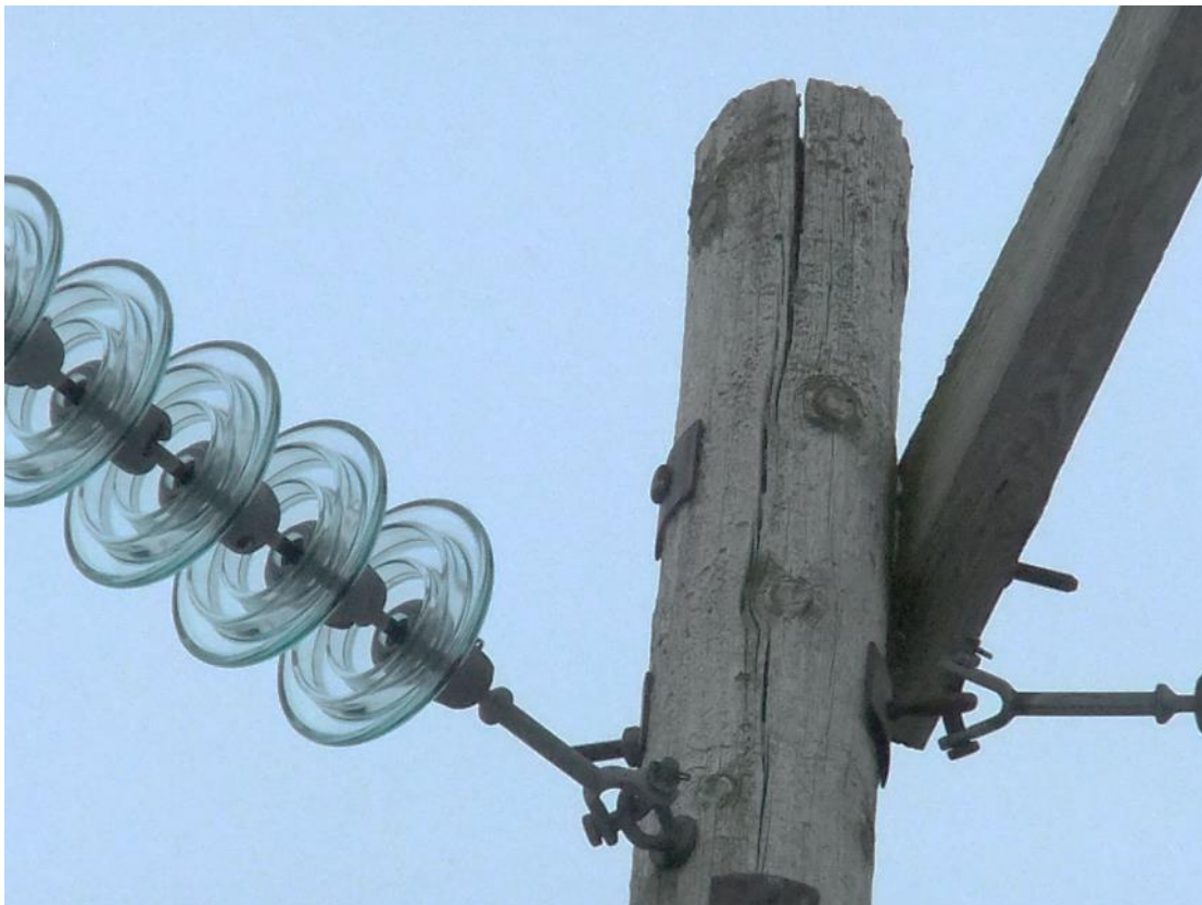
Figure 12 – Split Pole Top and Checking
