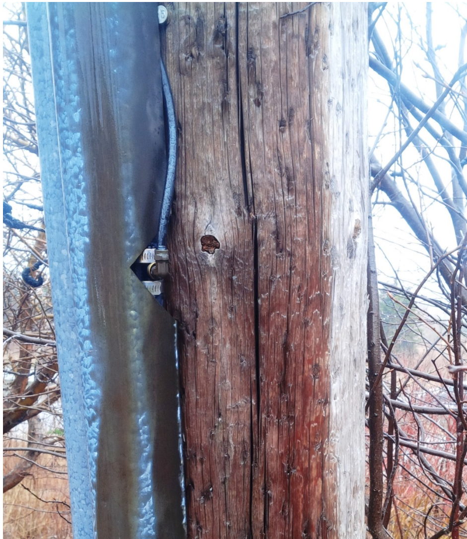
Figure 3 – GFS-02 Main Trunk Cracked Pole
