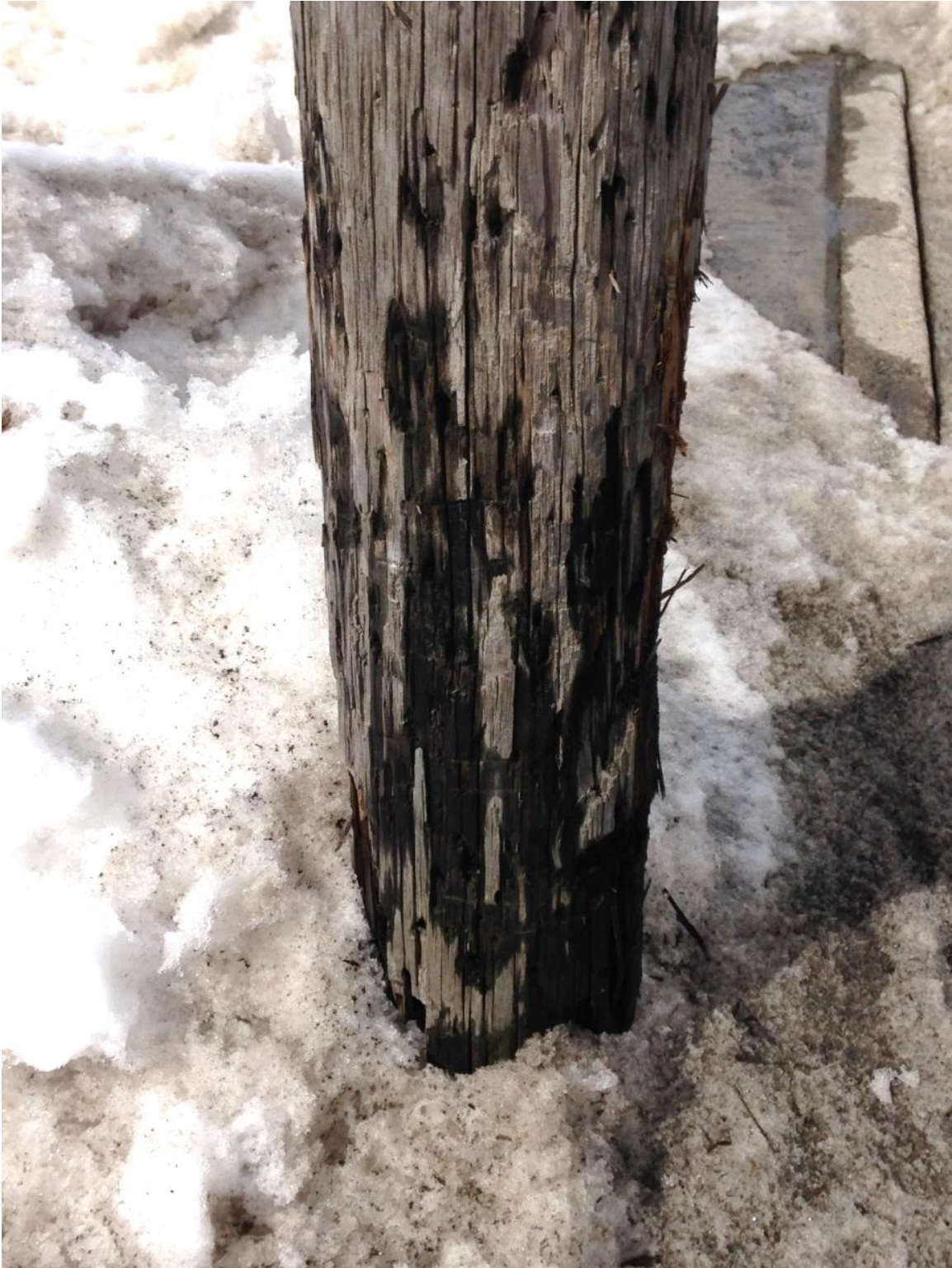
Figure 5 – Deteriorated Pole
