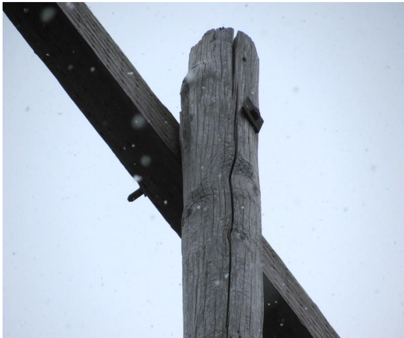
Figure 35 – Severe Check in Pole Top
