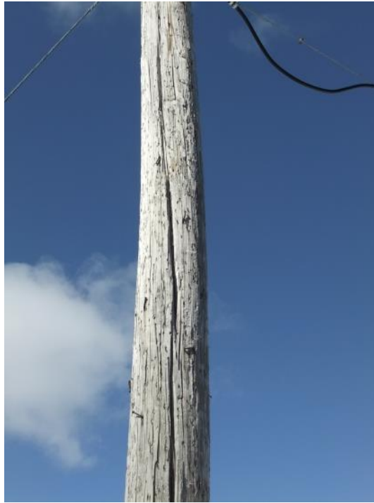
Figure 1 – Pole Checking
