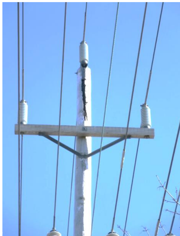
Figure 4 – Burned Pole
