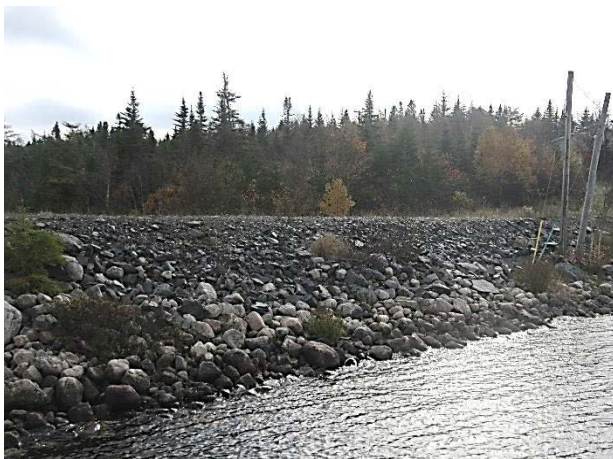
Figure 1 – Dam Riprap
