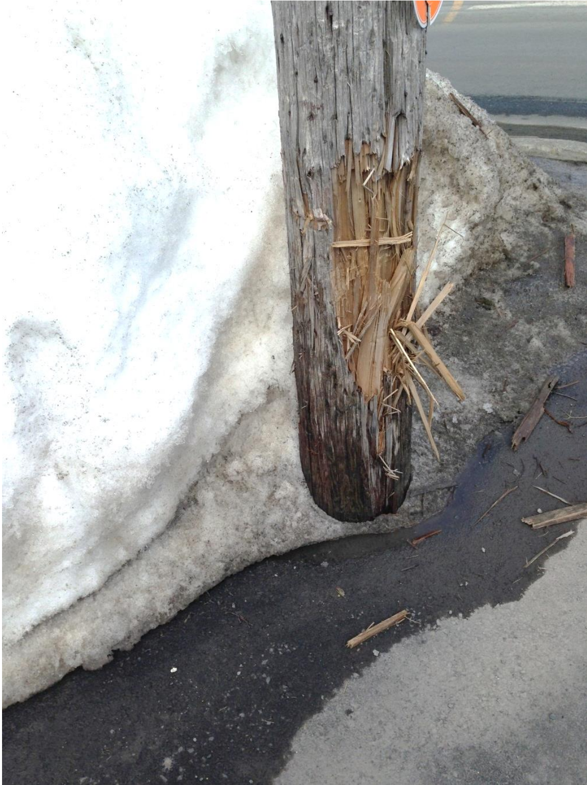
Figure 3 – Deteriorated Pole with Plow Damage
