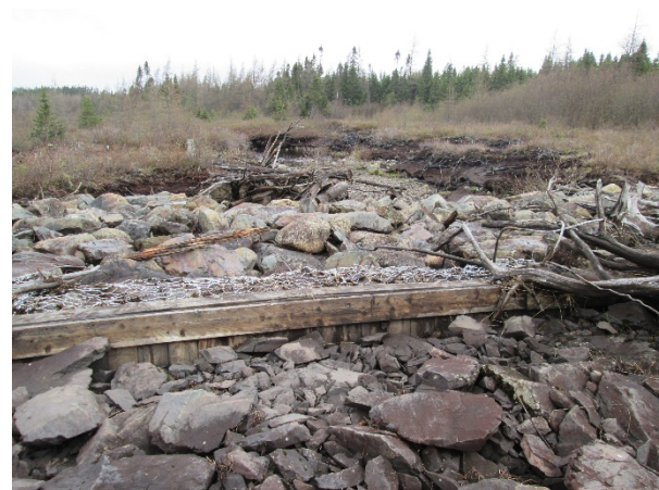
Figure 6 – Riprap Displacement and Downstream Erosion
