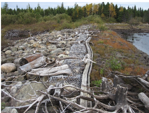
Figure 5 – Misaligned Core
