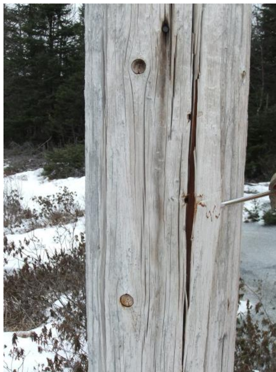
Figure 8 – Pole Shell Separation
