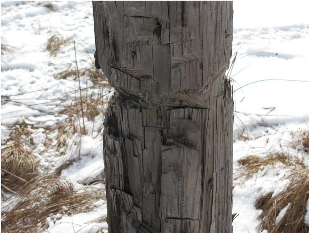
Figure 37 – Vandalism - Pole Damage
