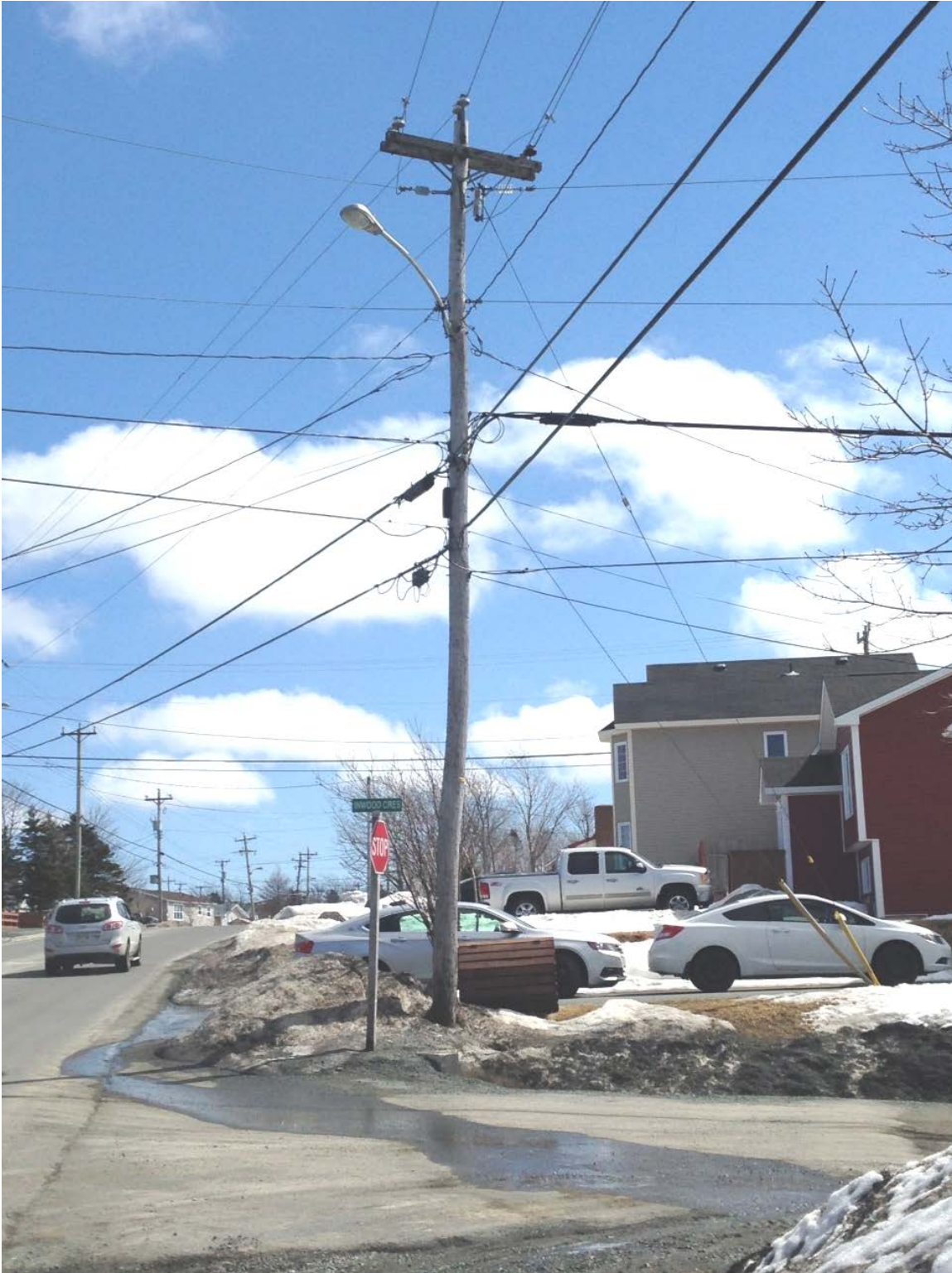
Figure 1 – Deteriorated Pole with Notable Bend and Obsolete Hardware
