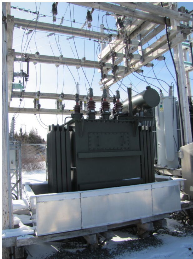
Figure 4: Existing VIC-T2 Spill Containment
