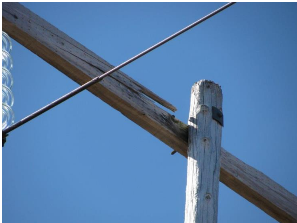
Figure 30 – Broken Crossarm
