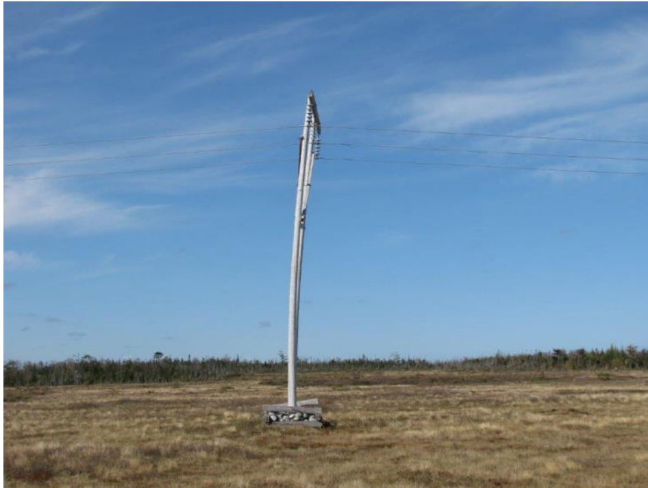
Figure 29 – Bent Structure
