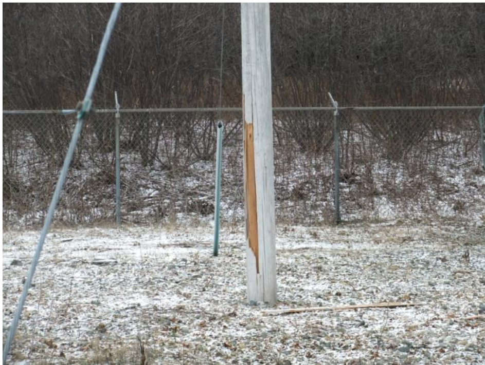
Figure 18 – Exposed Inner Wood
