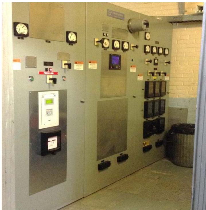
Figure 4 – Front of Switchgear
