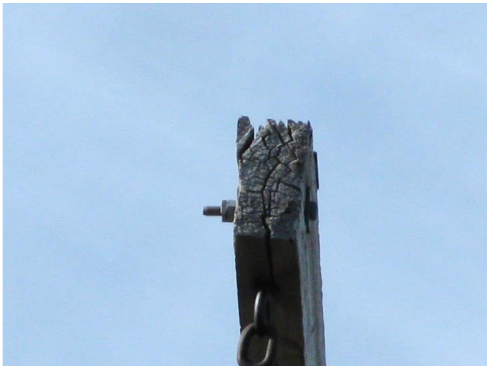
Figure 22 – Deteriorated Crossarm
