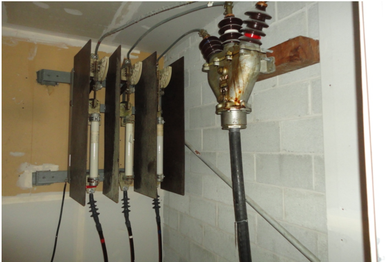
Figure 4: Credit Union Primary Feed and Disconnect Switch
