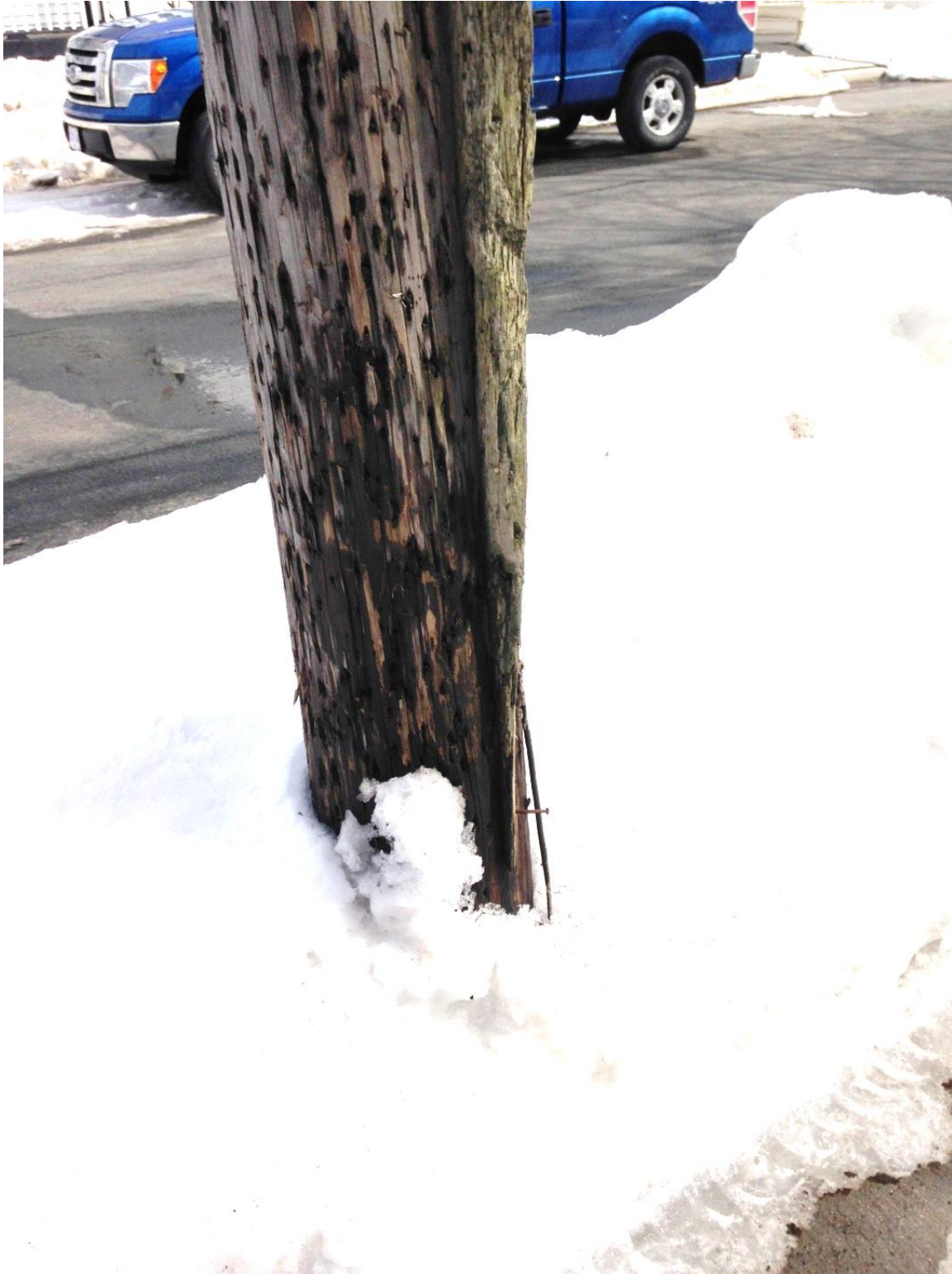
Figure 3 – Loss of Pole Diameter at Base
