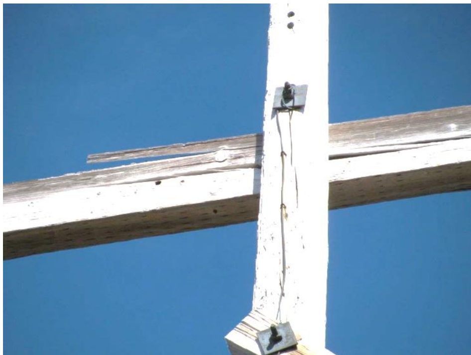
Figure 32 – Broken Crossarm
