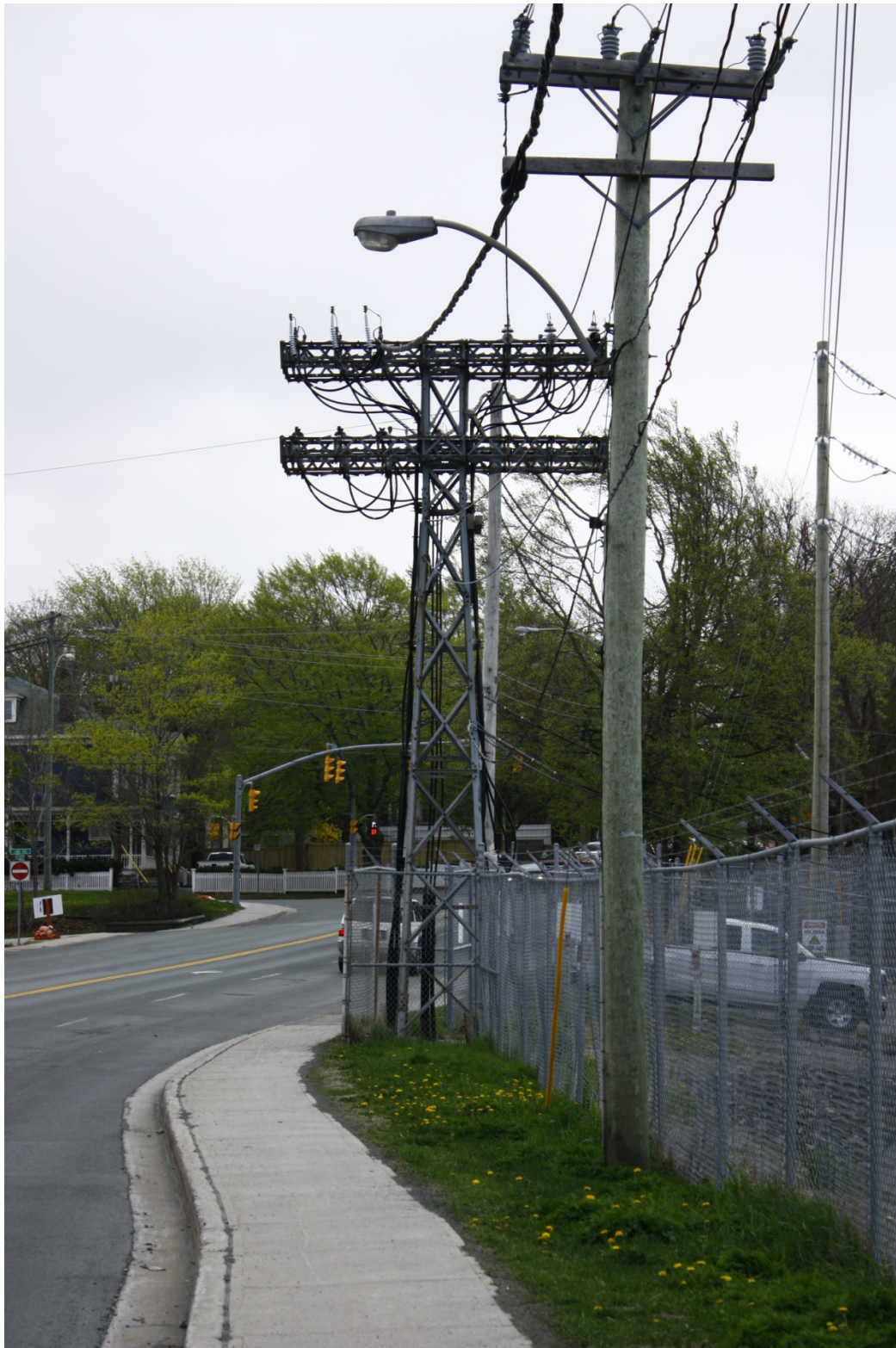
Figure 5: 4.16kV Steel Tower (King's Bridge Road)
