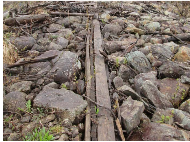
Figure 4 – Timber Core
