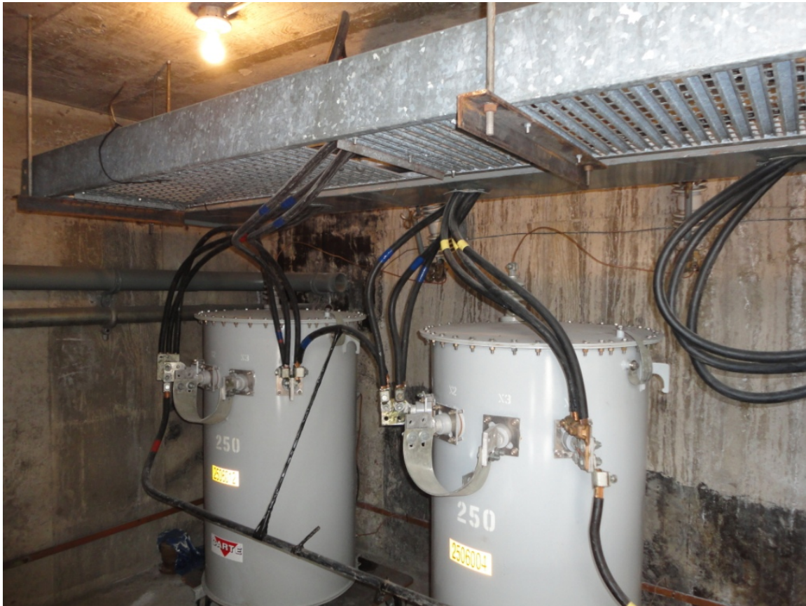
Figure 2: Battery Hotel Vault Transformers
