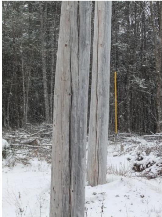
Figure 17 – Deep Pole Checking
