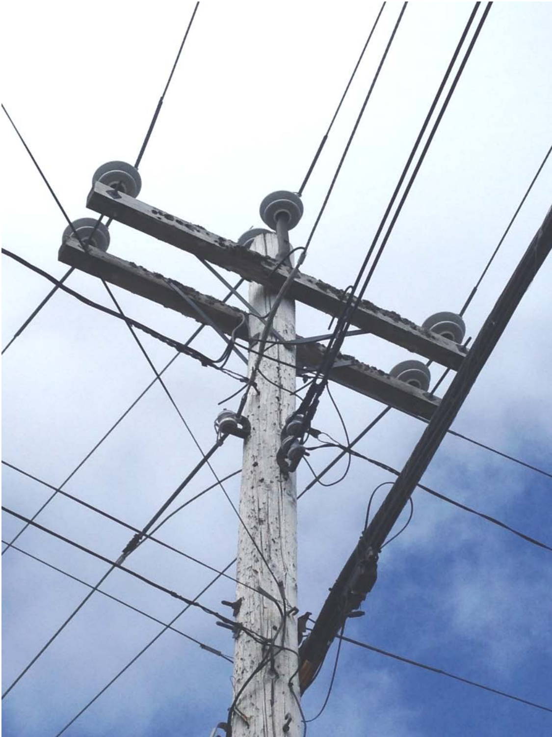
Figure 2 – Deteriorated Distribution Structure with 2-Piece Insulators
