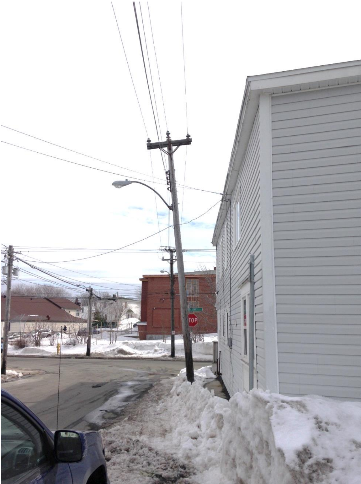
Figure 7 – Pole Leaning Towards Traffic
