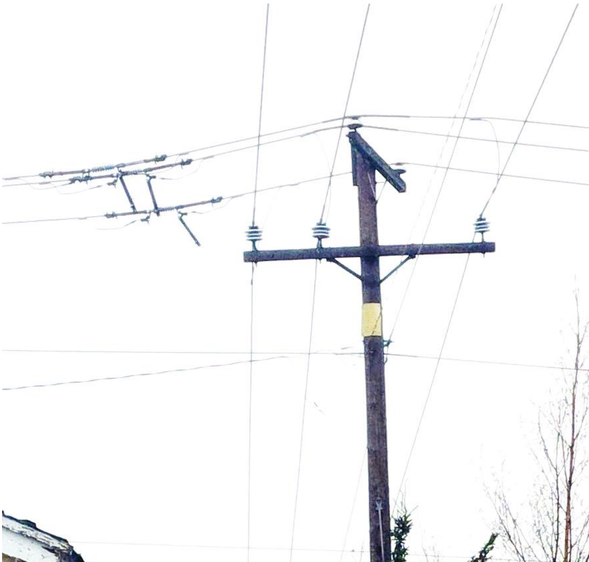
Figure 2 – GFS-02 Main Trunk Deteriorated Crossarm
