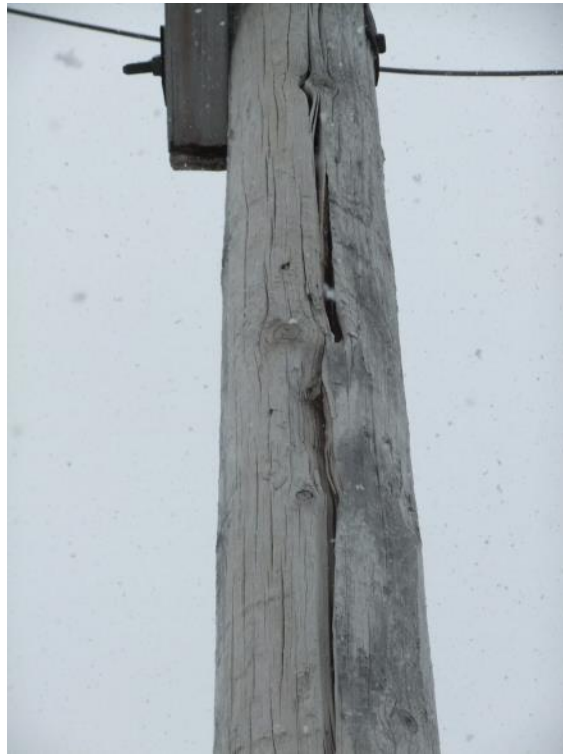
Figure 9 – Significant Pole Checking Due To Shell Separation
