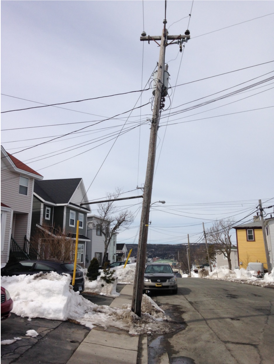
Figure 2 – Pole Leaning Towards Traffic
