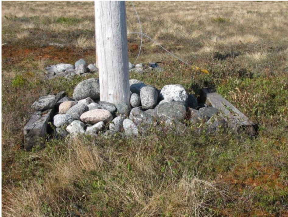
Figure 25 – Deteriorated Pole Crib
