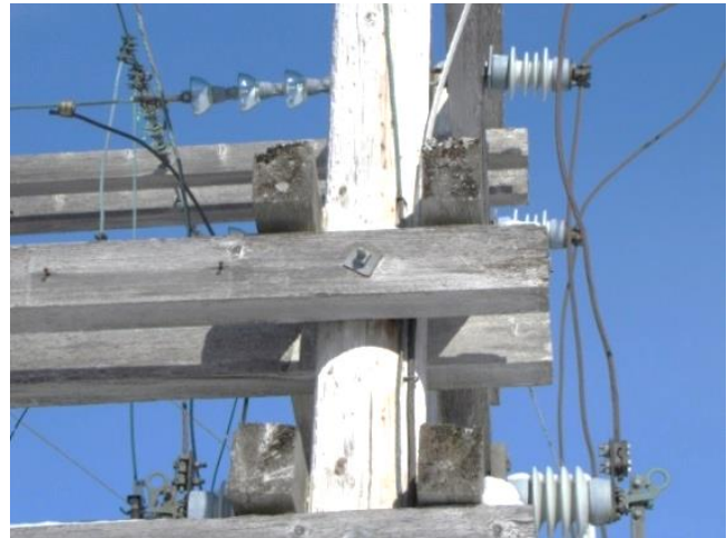
Figure 3: Deteriorated Cross Arms
