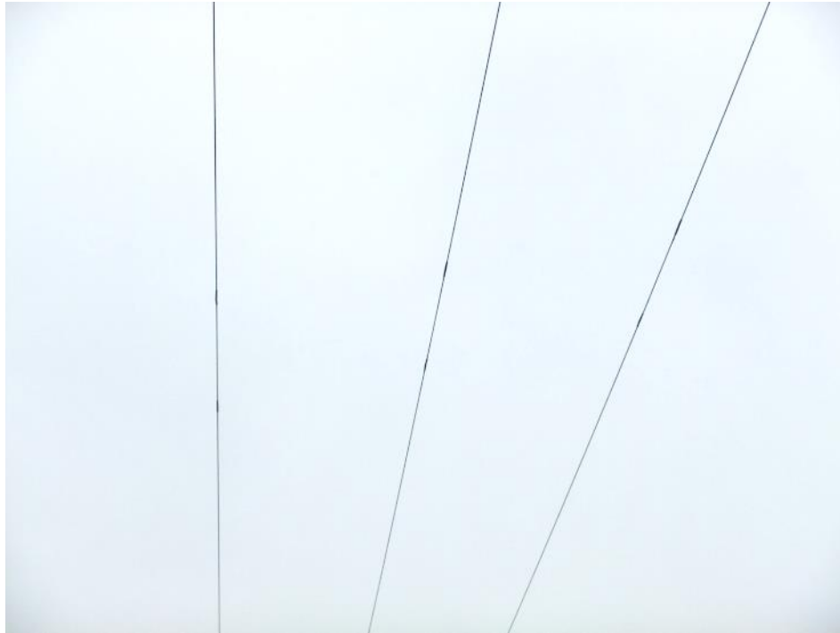
Figure 13 – Repairs to Conductor Due to Phase Contact Damage
