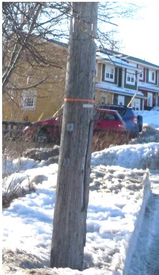
Figure 6 – Bolts Provide Temporary Repairs to Damaged Pole
