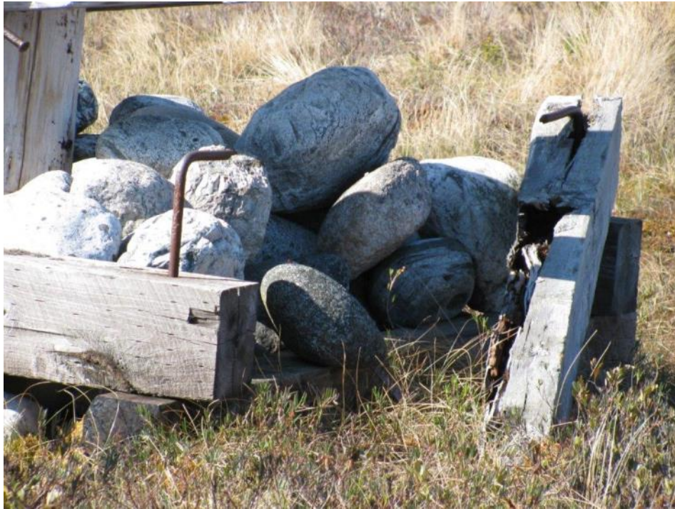
Figure 27 – Rock Ballast No Longer Contained
