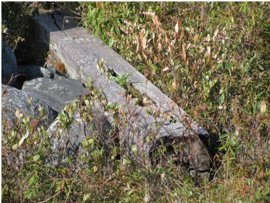
Figure 26 – Deteriorated Pole Crib Timber
