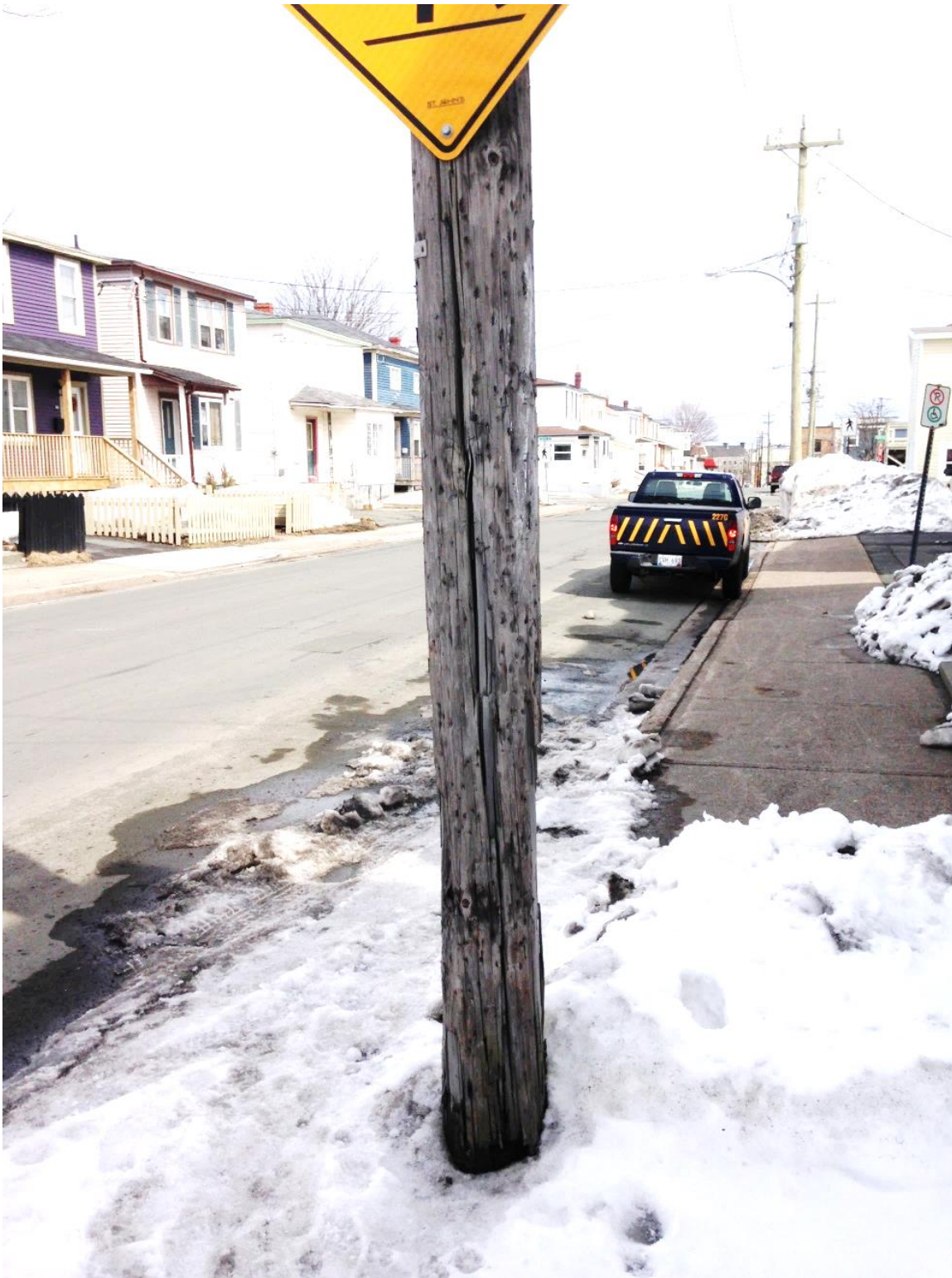
Figure 4 – Narrowed Pole Diameter at Base
