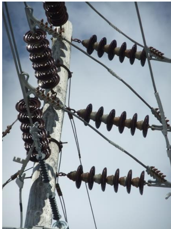
Figure 2 – 1950's Vintage Insulators and Hardware
