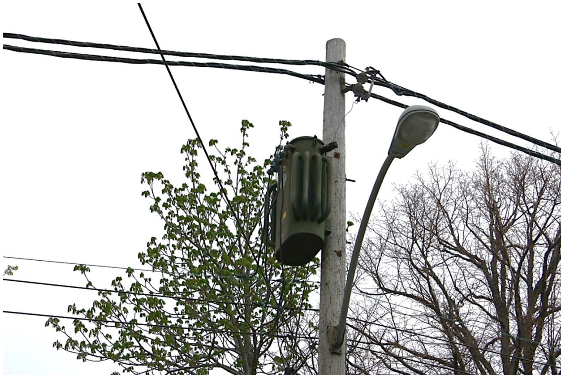
Figure 2: KBR-01 Non-Standard Transformer Connection
