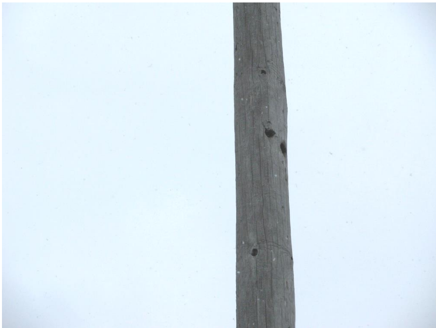
Figure 38 – Woodpecker Hole Damage
