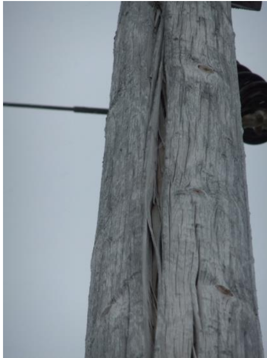
Figure 15 – Deep Checking Due to Shell Separation
