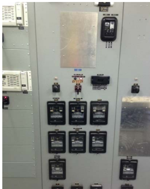
Figure 6: Existing GFS Control Building with Electromechanical Relays
