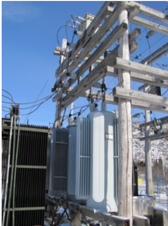
Figure 1: Inadequate Clearances
