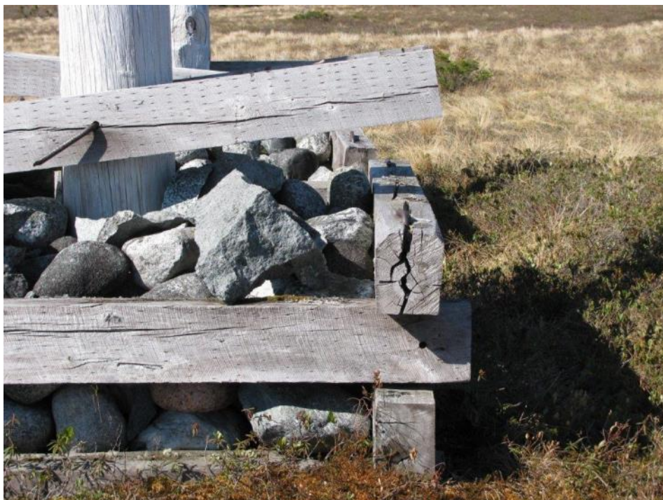
Figure 28 – Deteriorated Pole Crib Timber
