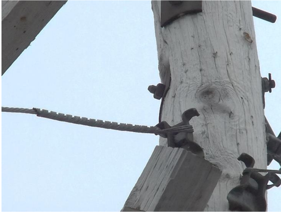
Figure 7 – Pole and Hardware Damage at Guy Wire Attachment
