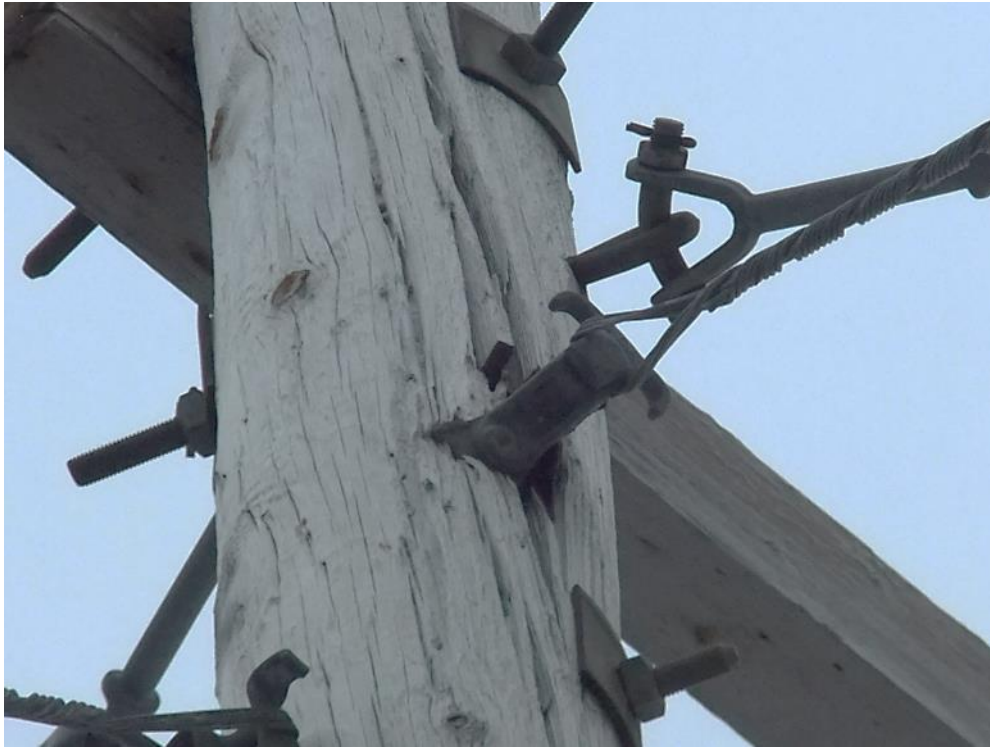
Figure 11 – Severe Pole Checking Due to Shell Separation
