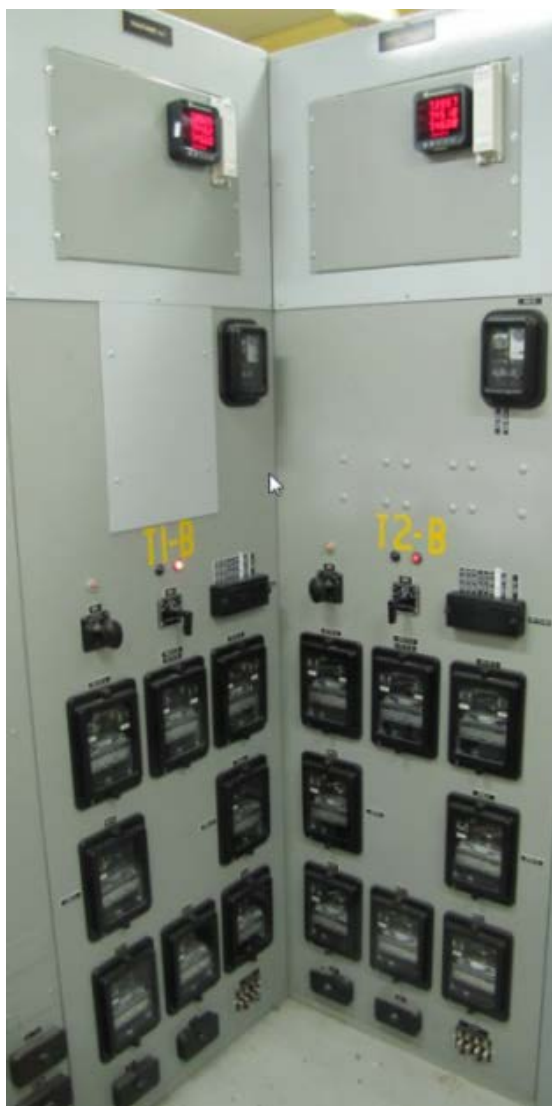
Figure 5: Existing VIR Control Building with Electromechanical Relays
