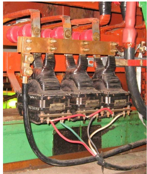
Figure 3 – Neutral Current Transformers
