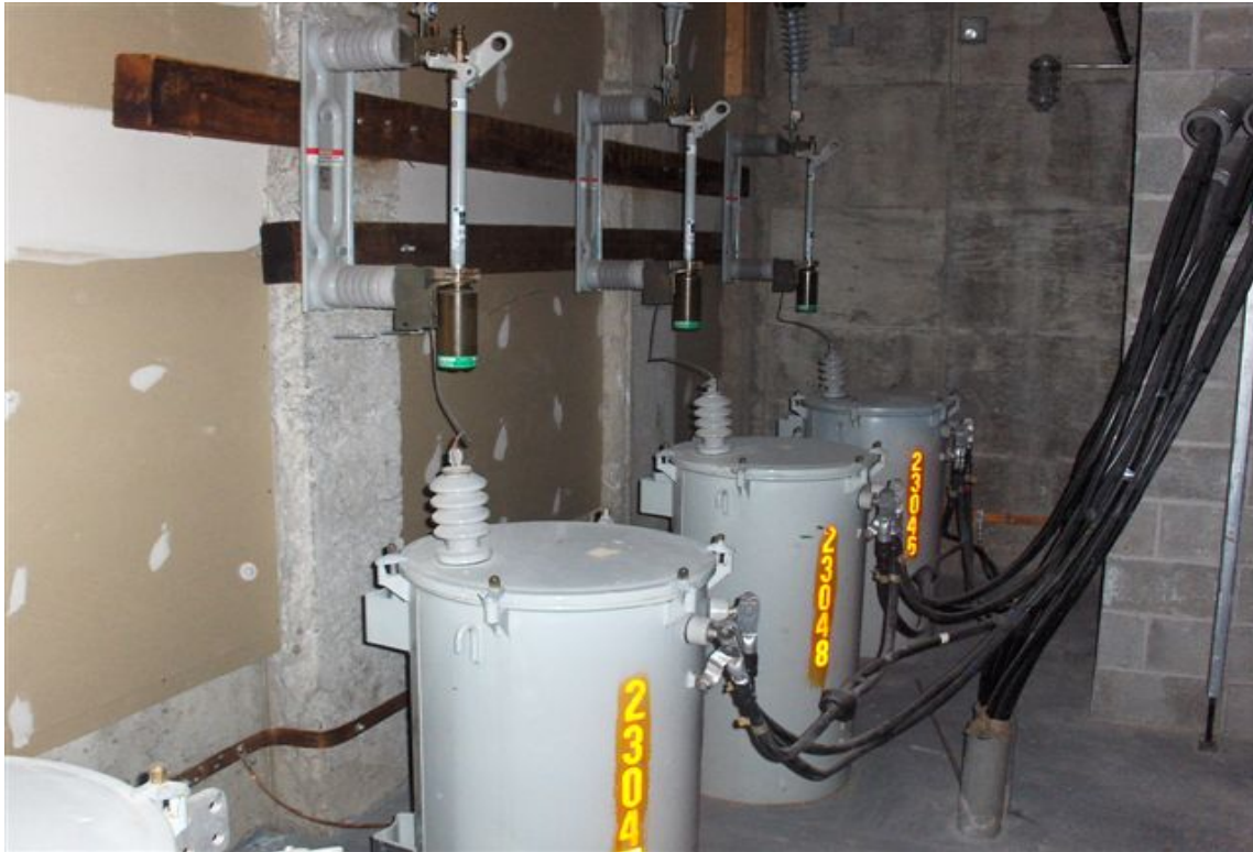
Figure 7: City Hall Annex Pole Mount Transformers and Cutouts
