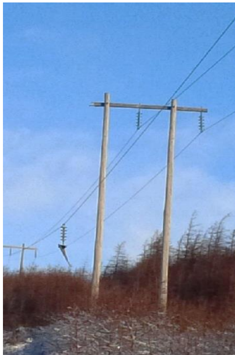
Figure 36 – Damage Resulting from Rotten Crossarm
