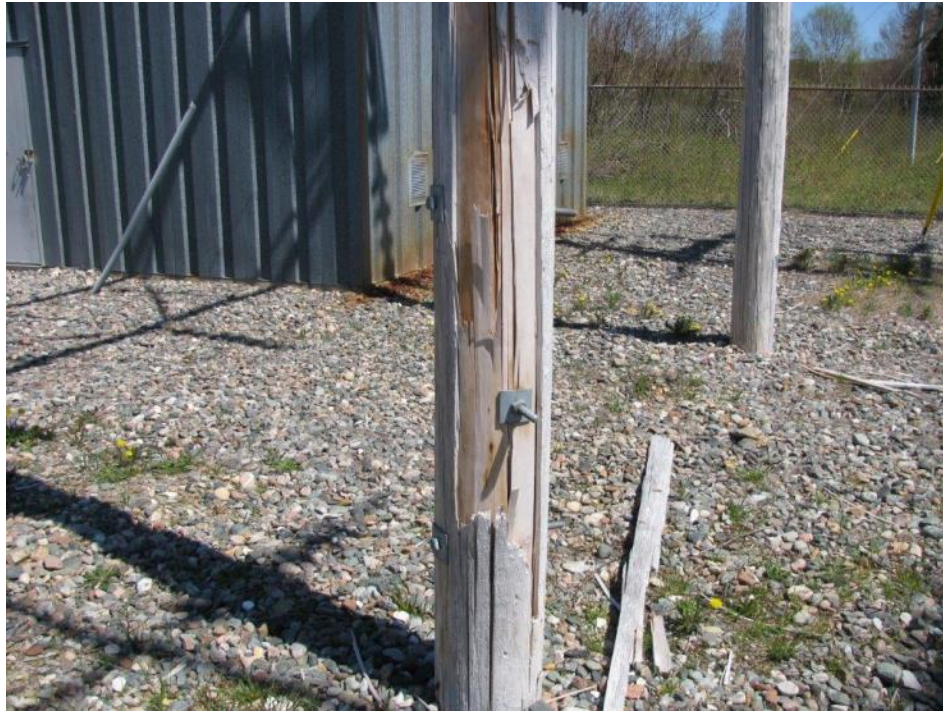
Figure 23 – Bolts Keeping Broken Pole Together
