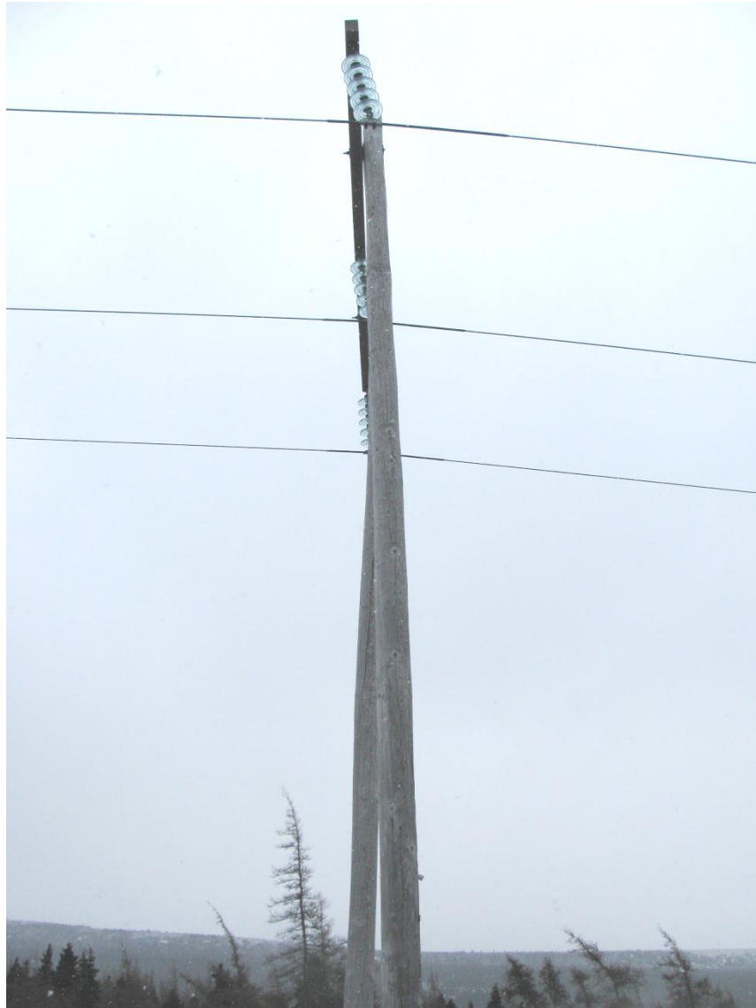
Figure 41 – Twisted Structure
