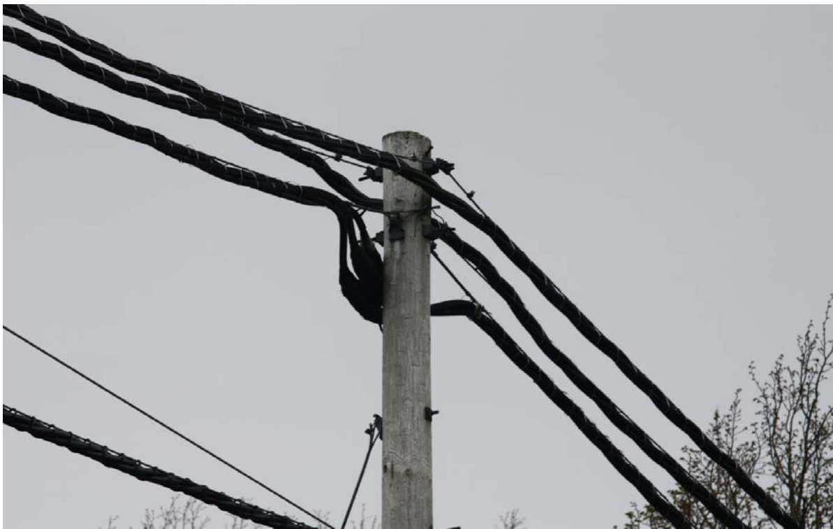
Figure 10: Aerial Cable Splices (King's Bridge Road)
