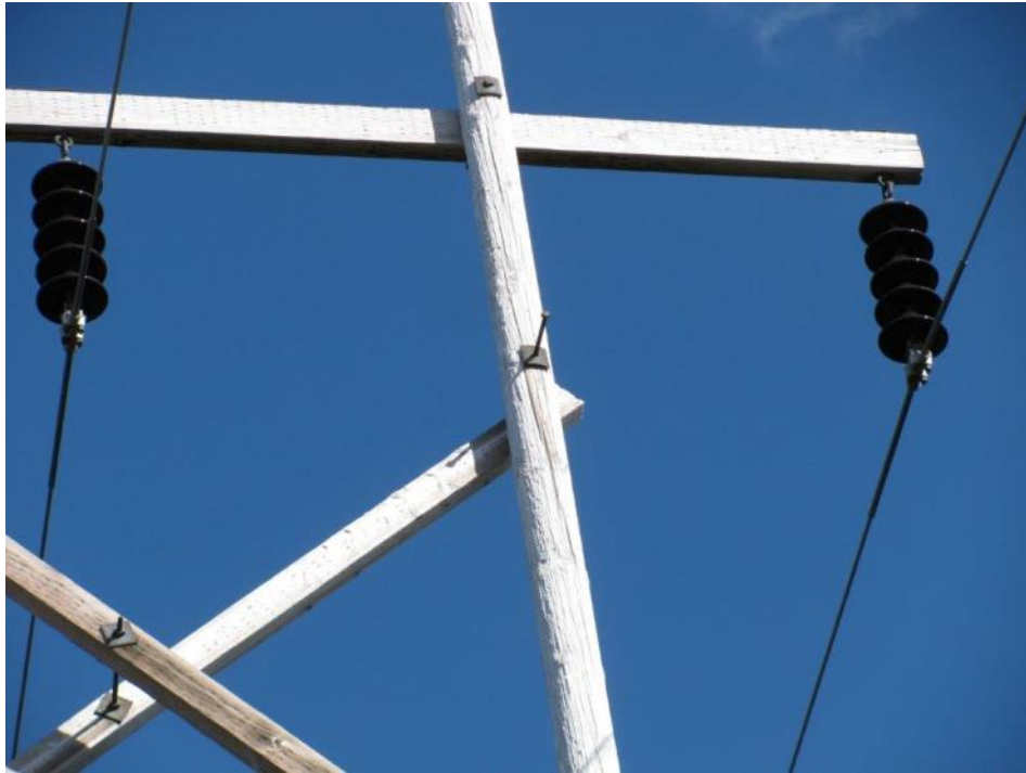
Figure 31 – Bolt No Longer Securing Cross Brace
