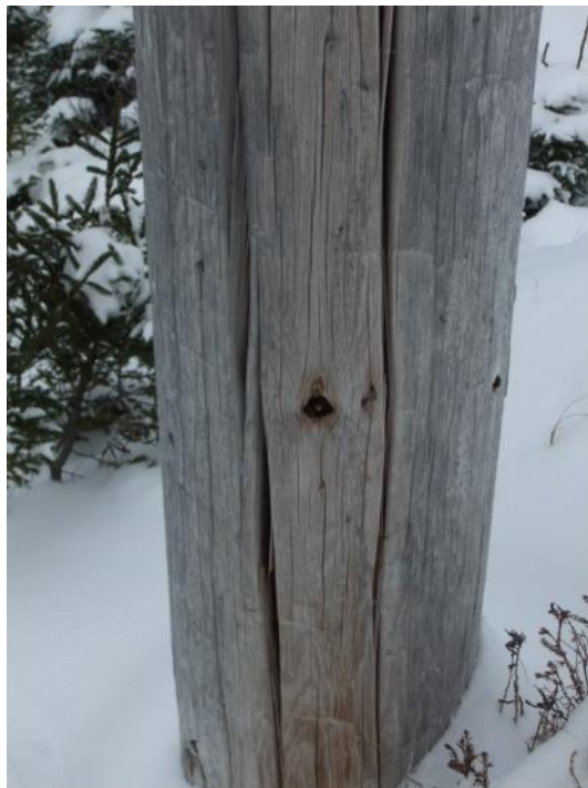
Figure 16 – Pole Shell Separation
