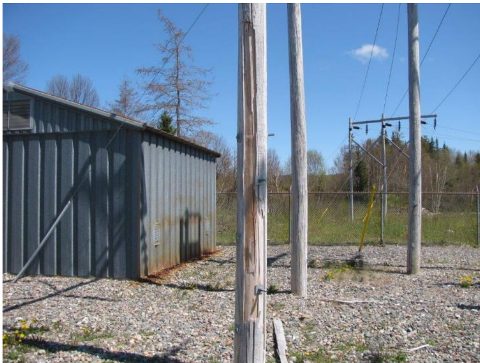
Figure 24 – Bolts Keeping Broken Pole Together
