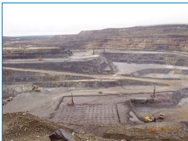
Mining activity at IOC's Luce Pit
