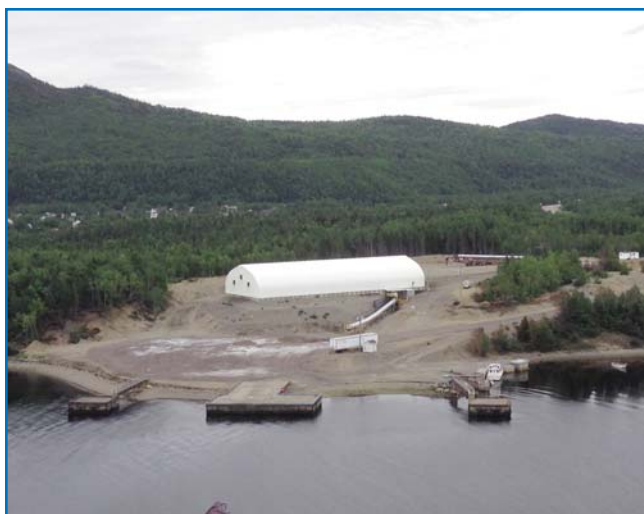
Rambler's concentrate storage shed at Goodyear's Cove
