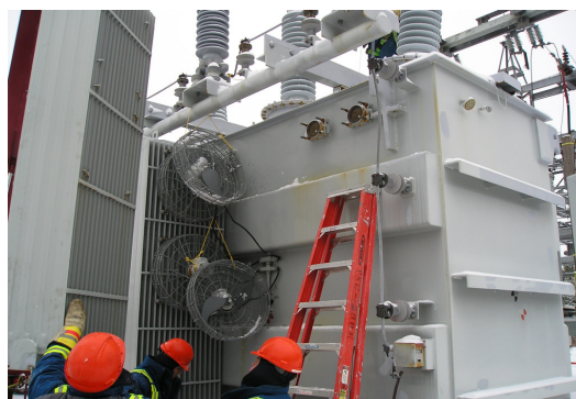
Figure 4: Radiators being replaced at Bottom Waters Terminal Station
