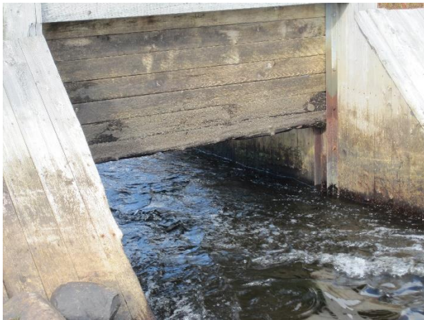
Figure 9 – Deteriorated Gate
