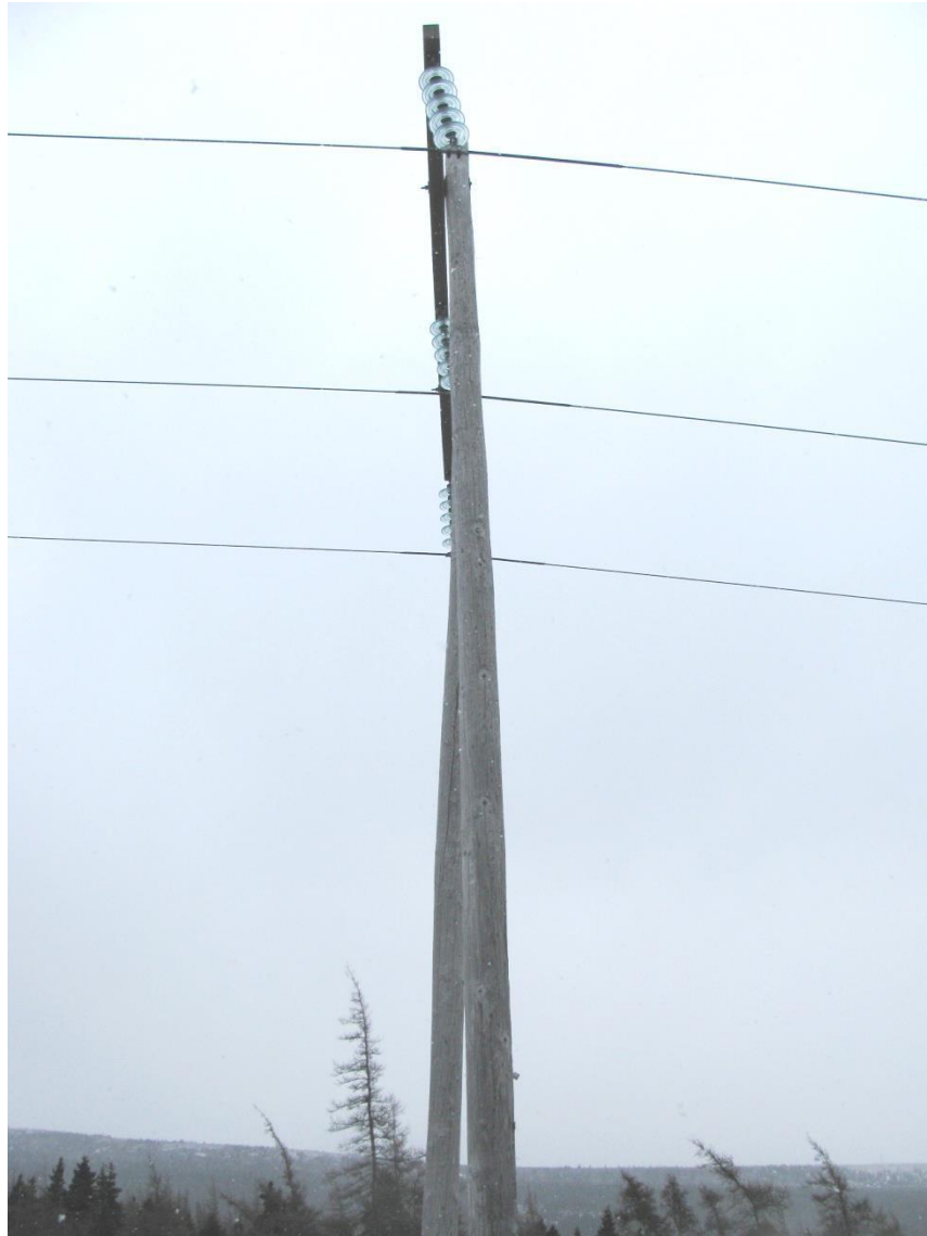
Figure 18 – Twisted Structure
