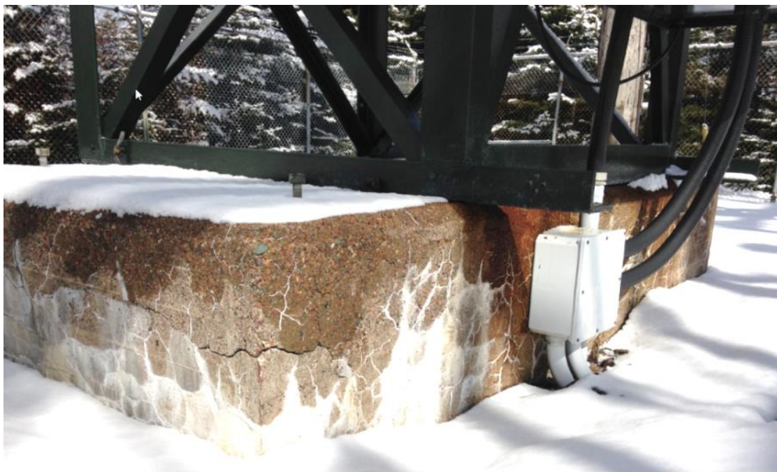
Figure 3: Deteriorated Foundation
