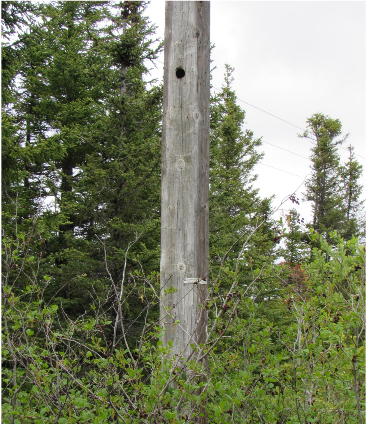
Figure 3 – Pole with Woodpecker Hole
