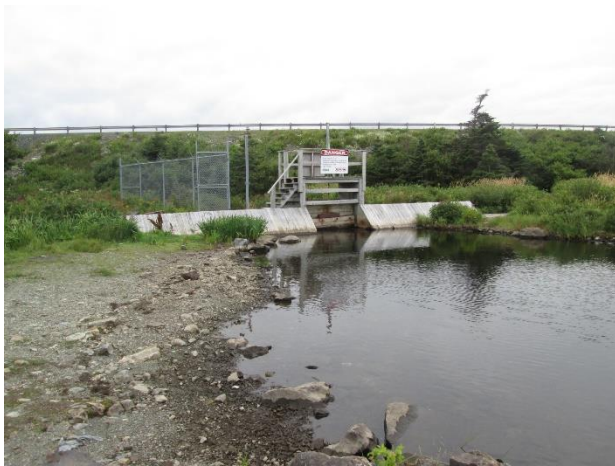
Figure 7 – Three Arm Pond Dam
