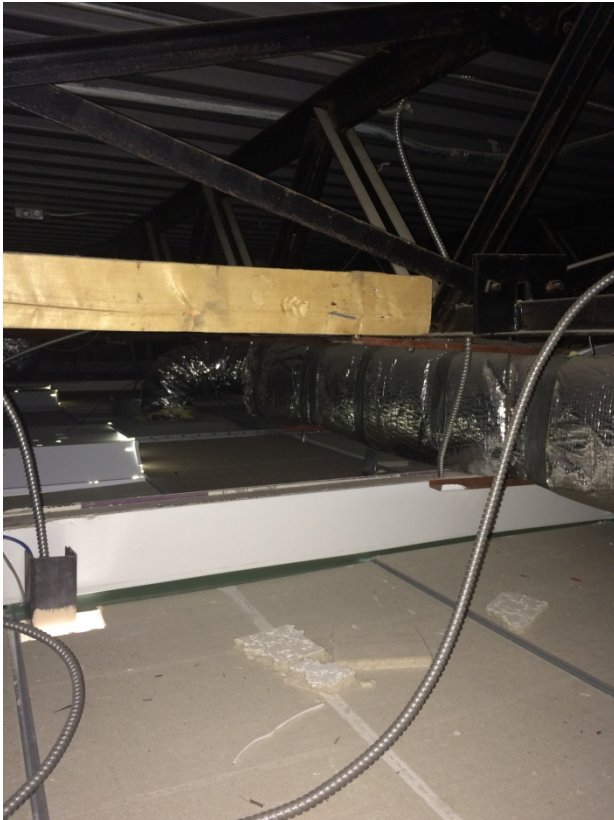
ROOF TOP HEAT PUMP RETURN/SUPPLY DISTRIBUTION
