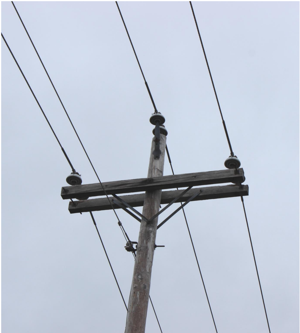
Figure 1 – Deteriorated Crossarm
