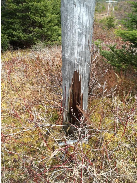
Figure 6 – Deteriorated Pole
