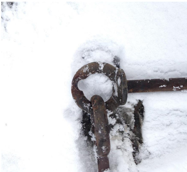
Figure 11 – Worn Ball Link Eye Bolt Recently Removed
