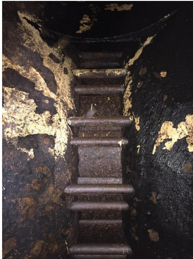
Figure 2 - G3 Scroll Case and Wicket Gates
