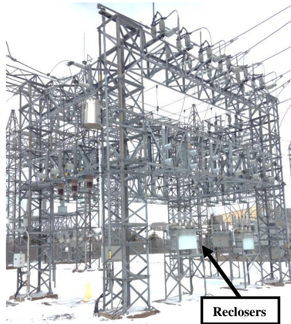
Figure 4: Hydraulic Reclosers
