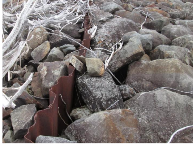
Figure 4 – Steel Spillway Core
