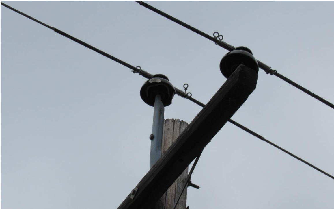
Figure 4 – Damaged Insulators
