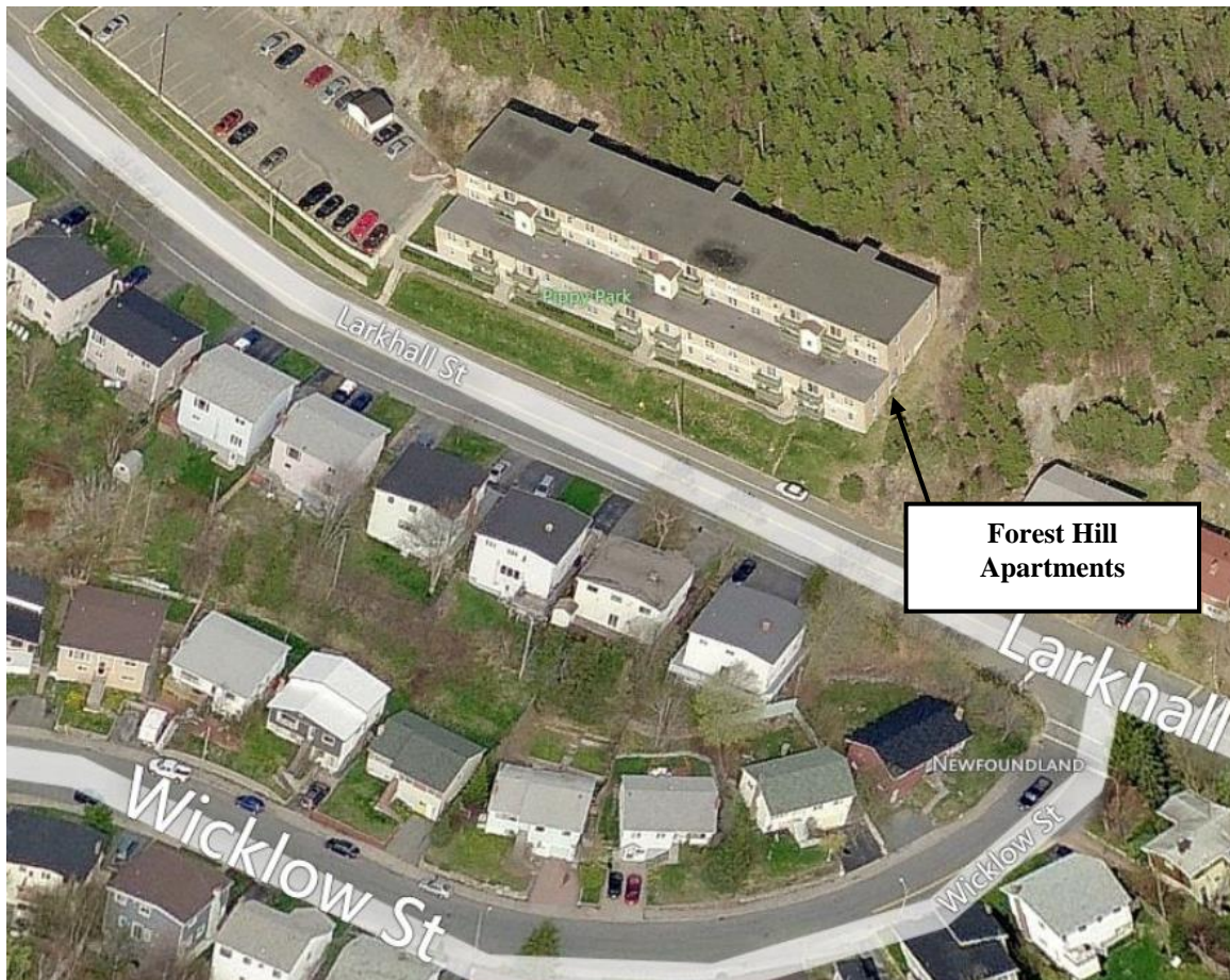
Figure 1: Forest Hill Apartments Vault Location
