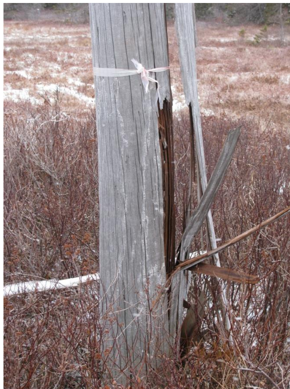
Figure 17 – Outer Shell Layer Separation
