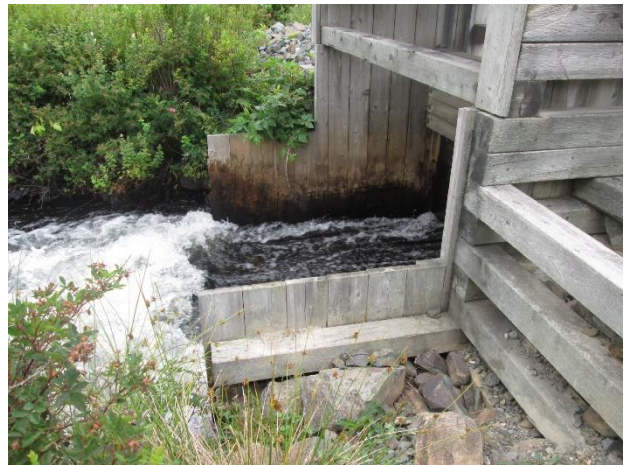
Figure 10 – Deteriorated Timbers
