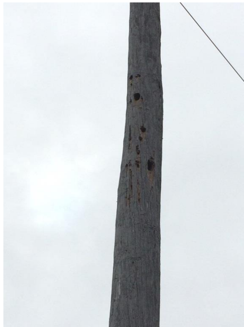
Figure 7 – Woodpecker Holes in Pole
