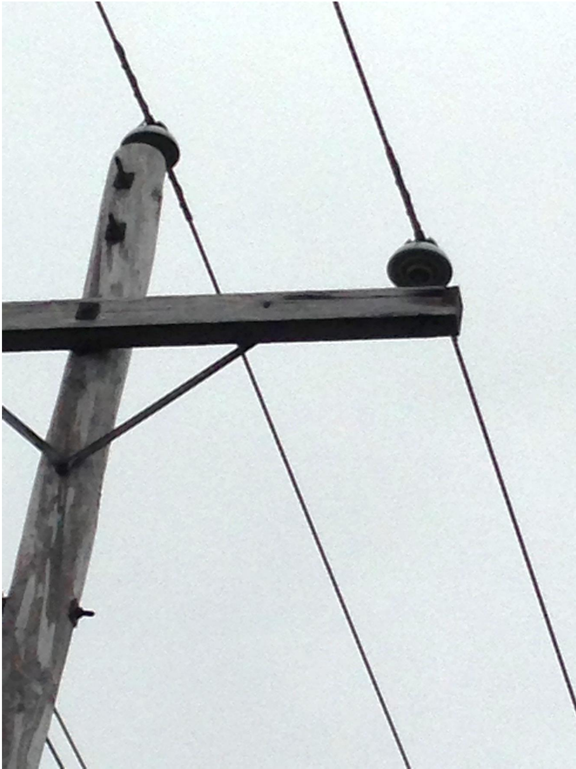
Figure 4 – Deteriorated Crossarm
