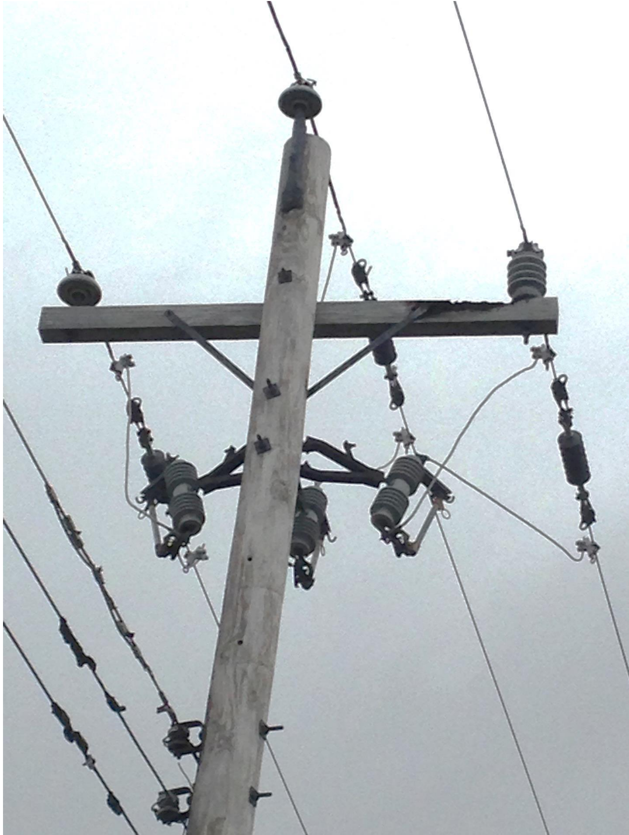
Figure 4 – Deteriorated Crossarm
