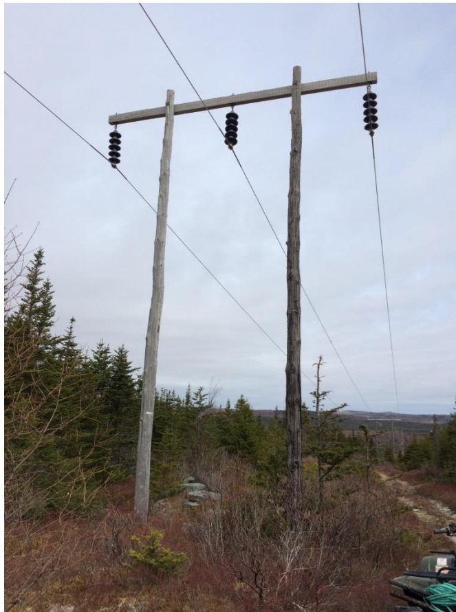
Figure 9 – Original Structure Without Crossbracing
