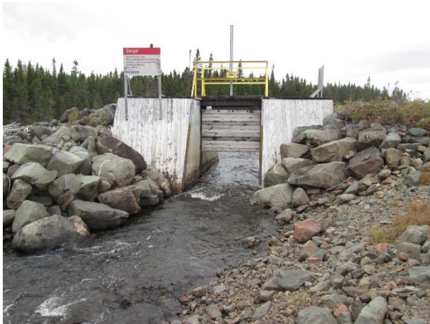
Figure 1 – Outlet Structure (Upstream)
