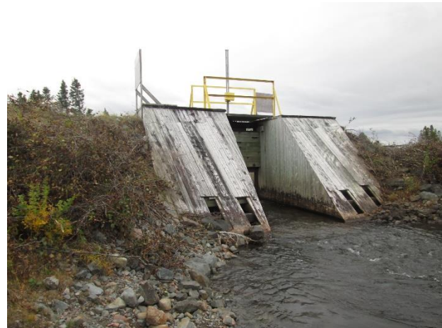
Figure 2 – Outlet Structure (Downstream)
