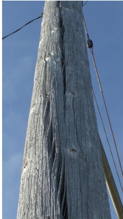
Figure 1 – Pole Checking
