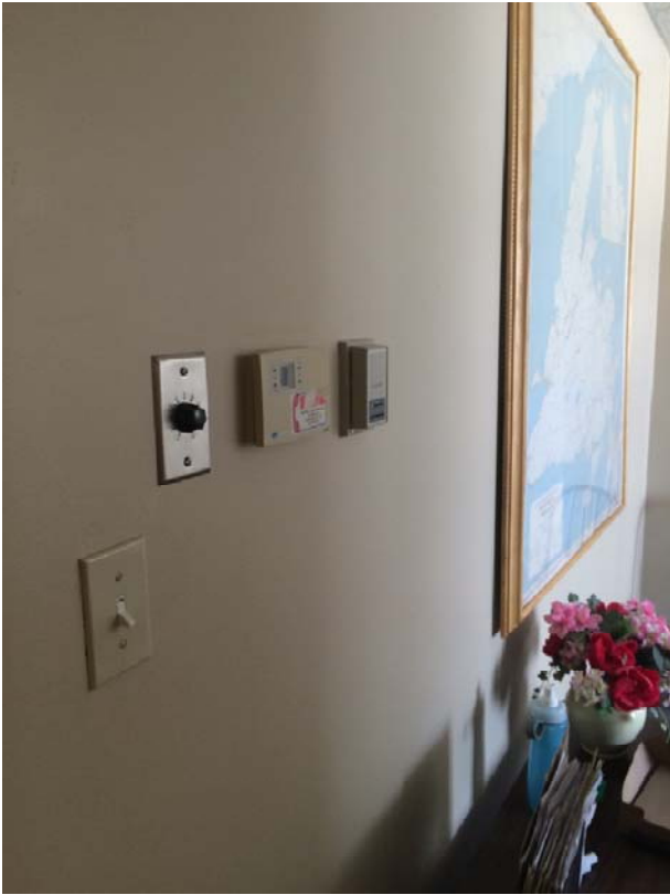
HEAT PUMP AND BASEBOARD HEAT THERMOSTATS
