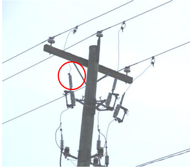
Figure 8: Current Limiting Fuses In Service
