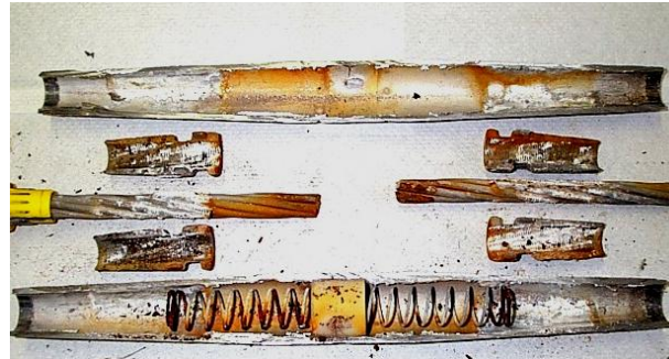
Figure 10: Disassembled Automatic Sleeve Showing Corrosion
