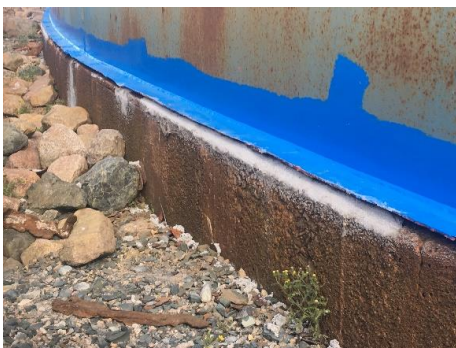
Figure 3: View of concrete ring beam repairs.
