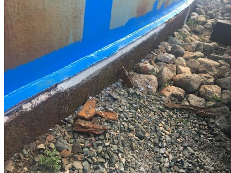
Figure 2: View of concrete ring beam repairs.
