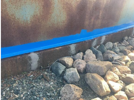
Figure 1: View of concrete ring beam repairs.
