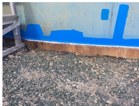
Figure 4: View of sealant applied to tank chine and ring beam interface.
