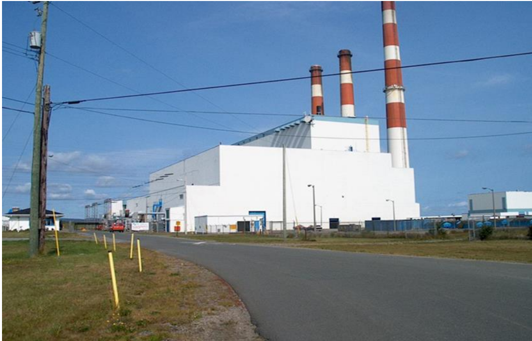
Figure 1: Holyrood Thermal Generating Station
