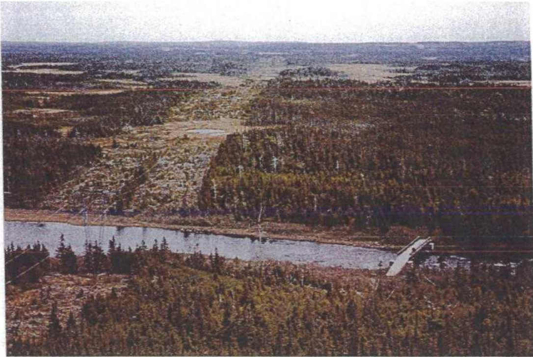
TL 202/TL 206 right of way with existing Hydro access bridge within the Bay Du Nord Wilderness Reserve
