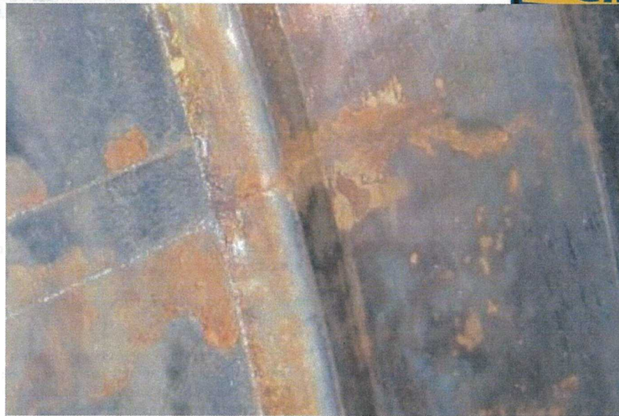
Figure 1: Exciter End Retaining Ring with Visible Cracks
