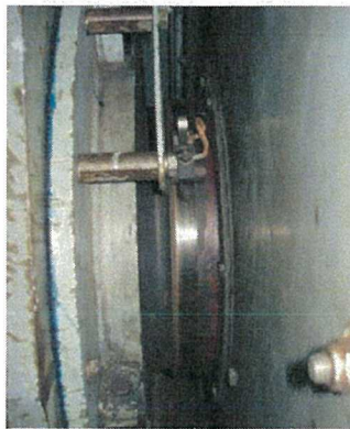
Rotor Shaft Earthing Brush
