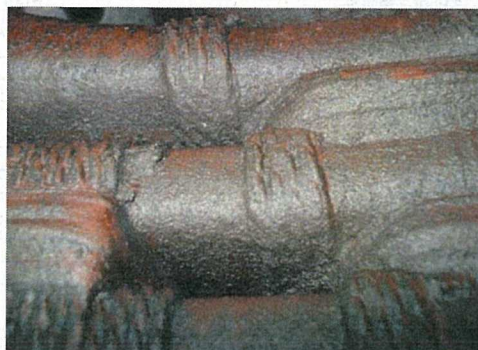
Contaminated Coils
