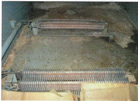
Anti Condensation Heaters
