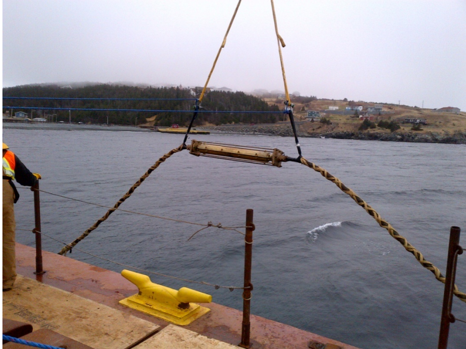
Photograph 6 – Placement of repaired cable onto sea bottom.
