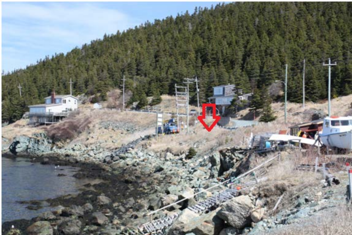
Figure 4 – Broad Cove Shoreline Termination Structure (arrow indicating proposed location of new structure)
