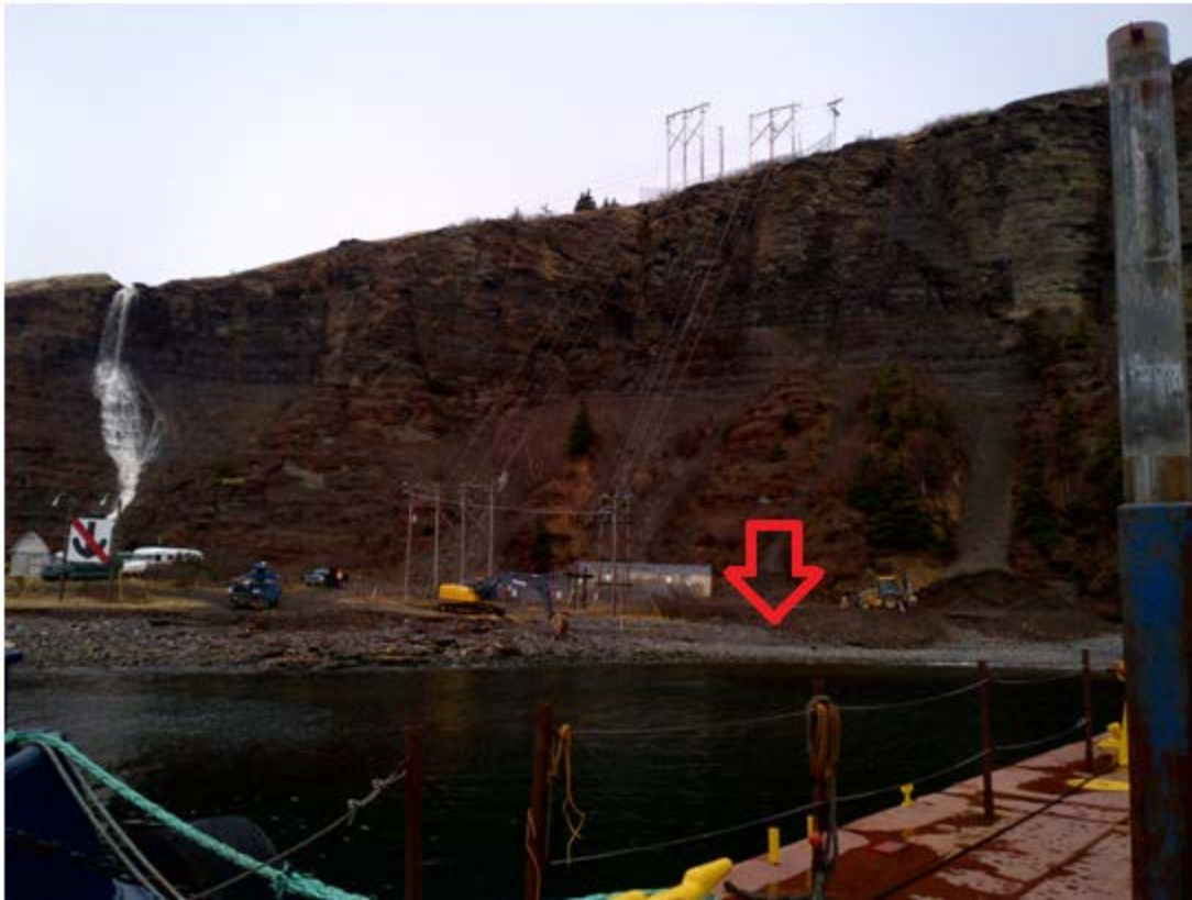
Figure 3 – Bell Island Onshore Termination and Distribution Structures (arrow indicating proposed location of new structure)
