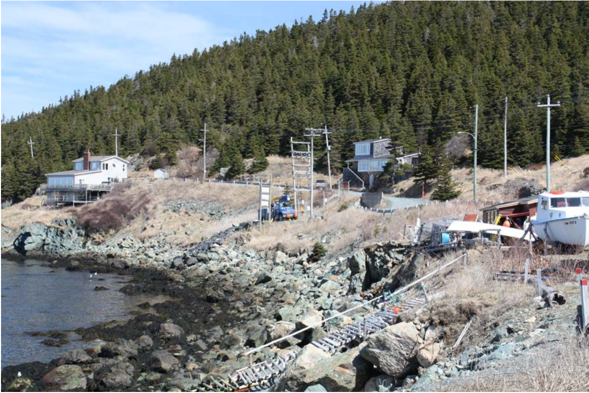
Figure 5 – View of Broad Cove Shoreline Termination Structure
