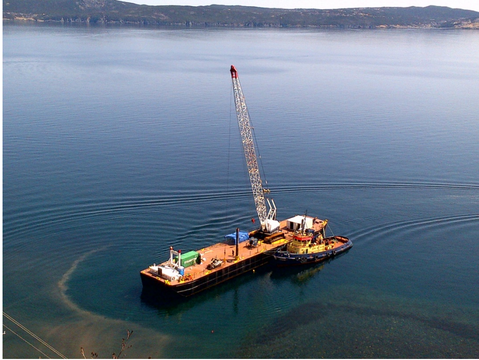
Photograph 1 – Cable repair vessels.
