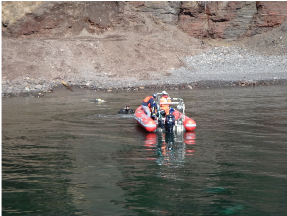
Photograph 8 – Divers installing cable protection (cast iron necklaces).
