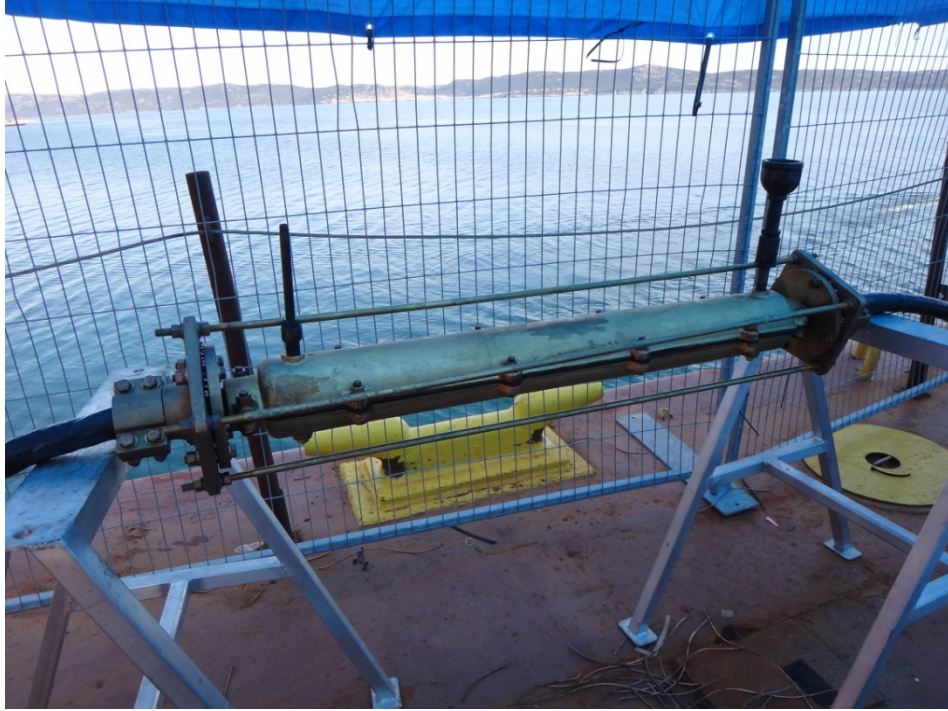
Photograph 5 – Completed submarine cable splice.
