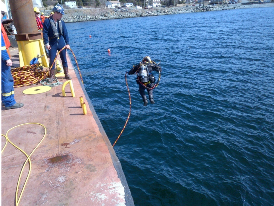
Photograph 2 – Diver leaving marine work platform.
