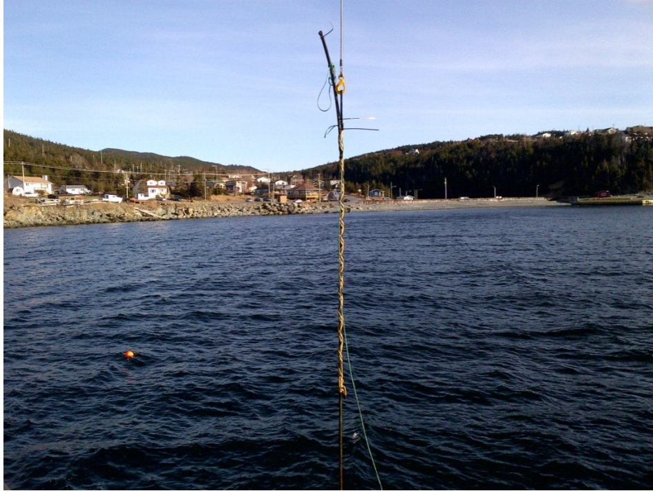
Photograph 3 – Cable retrieval to marine work platform.
