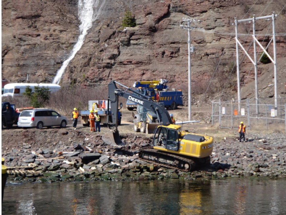
Photograph 7 – Shore approach excavation and trenching work at Bell Island.
