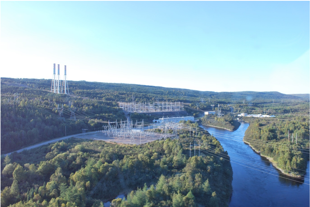
Figure 2: Bay d'Espoir Hydro Generating Station Site
