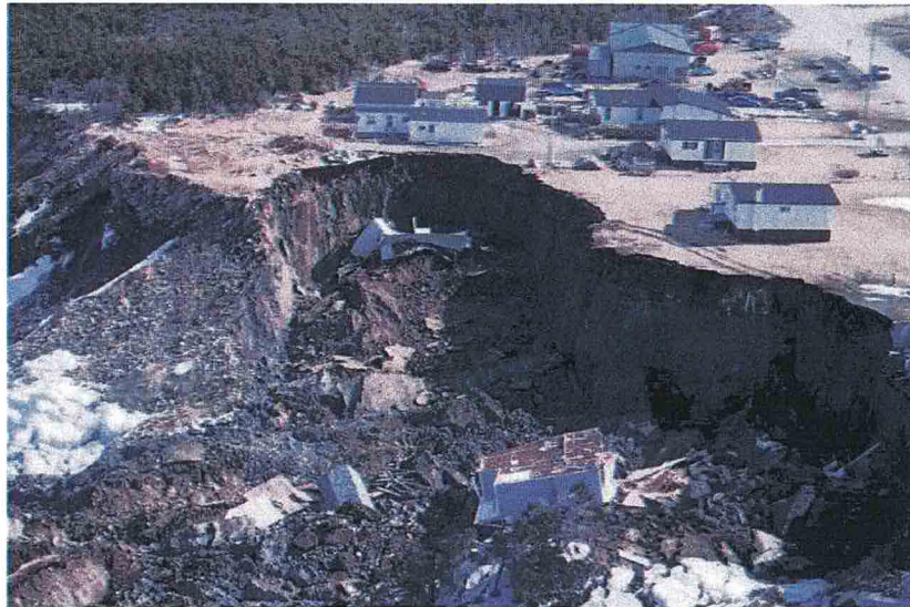
Figure 5: Results of Landslide in Daniel's Harbour 2007
