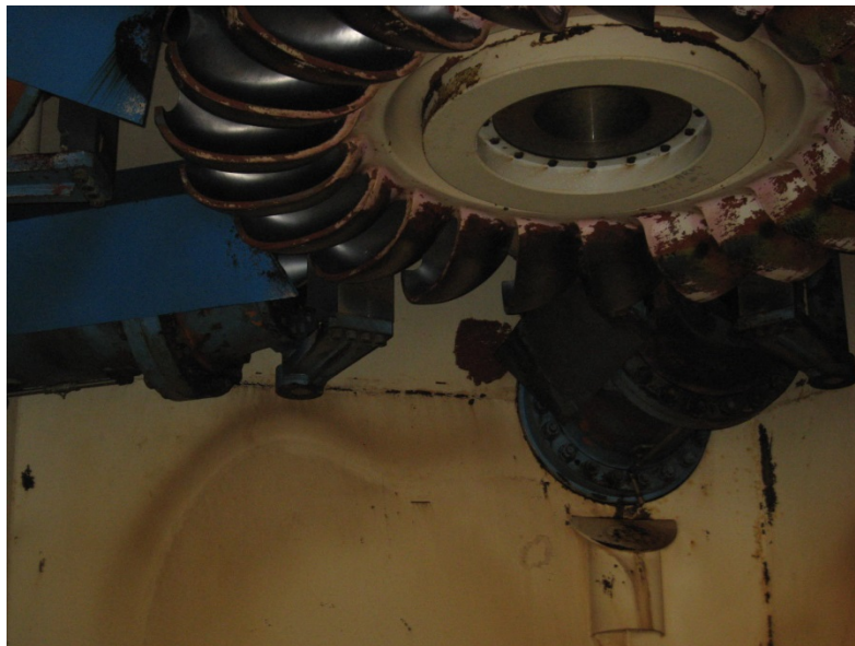
Figure 2: Cat Arm Pelton Turbine (Runner and jets)
