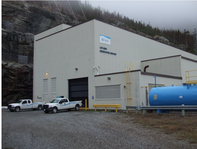
Figure 1: Cat Arm Hydro Generating Station
