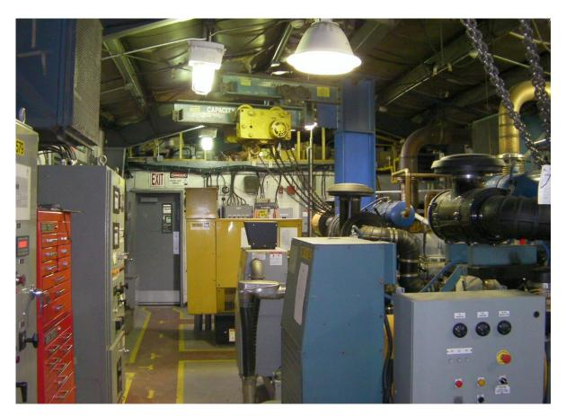
Figure 2: Black Tickle – Diesel Generators in Powerhouse
