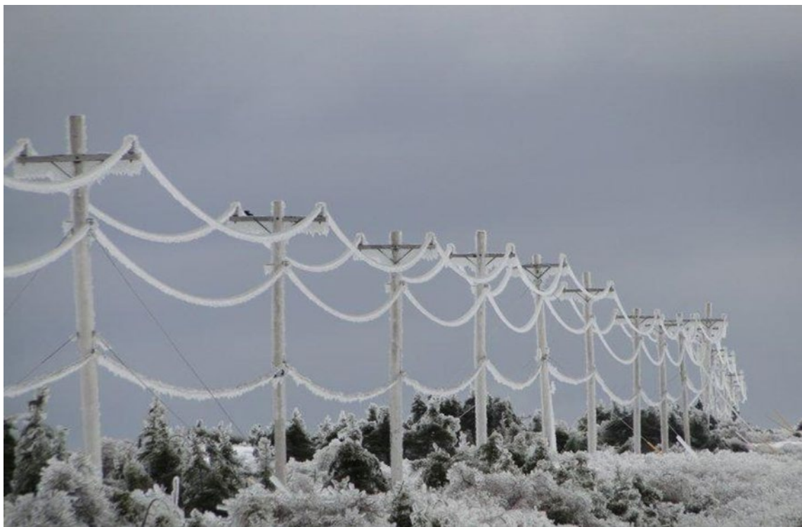
Figure 9: Ice loading on Newfoundland Power lines during 2010 ice storm
