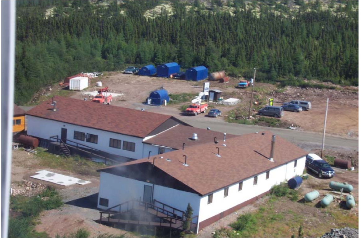
Normore – Decommissioned tankage from Marine Depot - Cartwright
