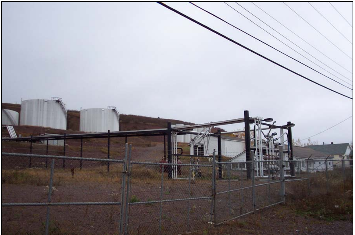
Irving – Marine Terminal – Botwood - Decommissioned
