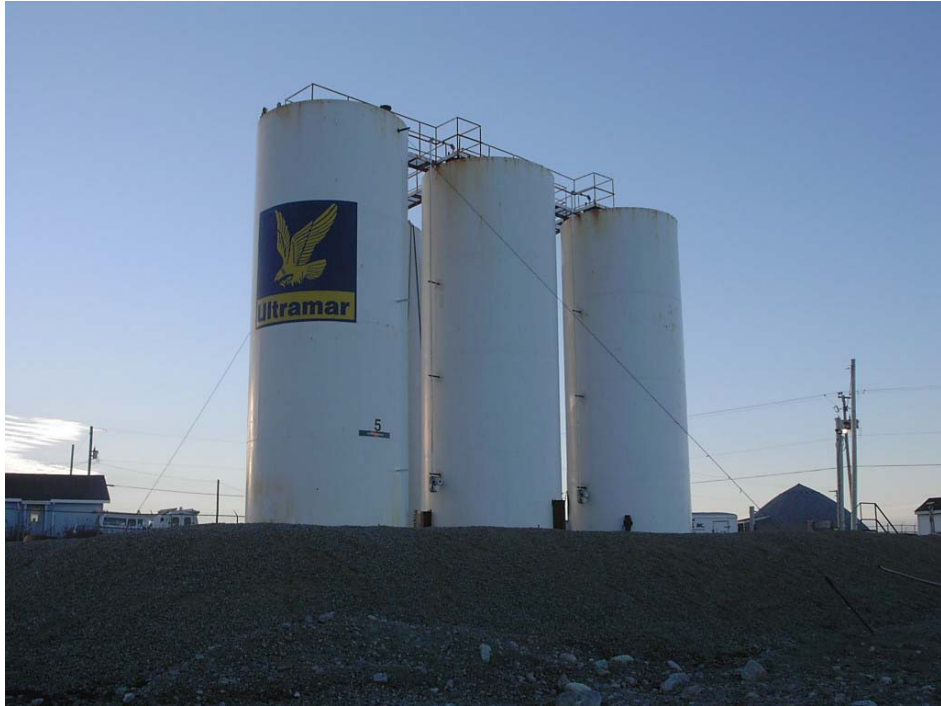
Ultramar – Bulk Plant – Port aux Basques – Tankage
