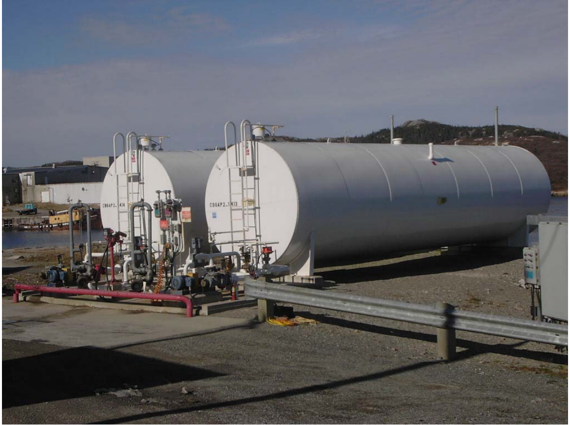
Western Petroleum - Bulk Plant – Burgeo
