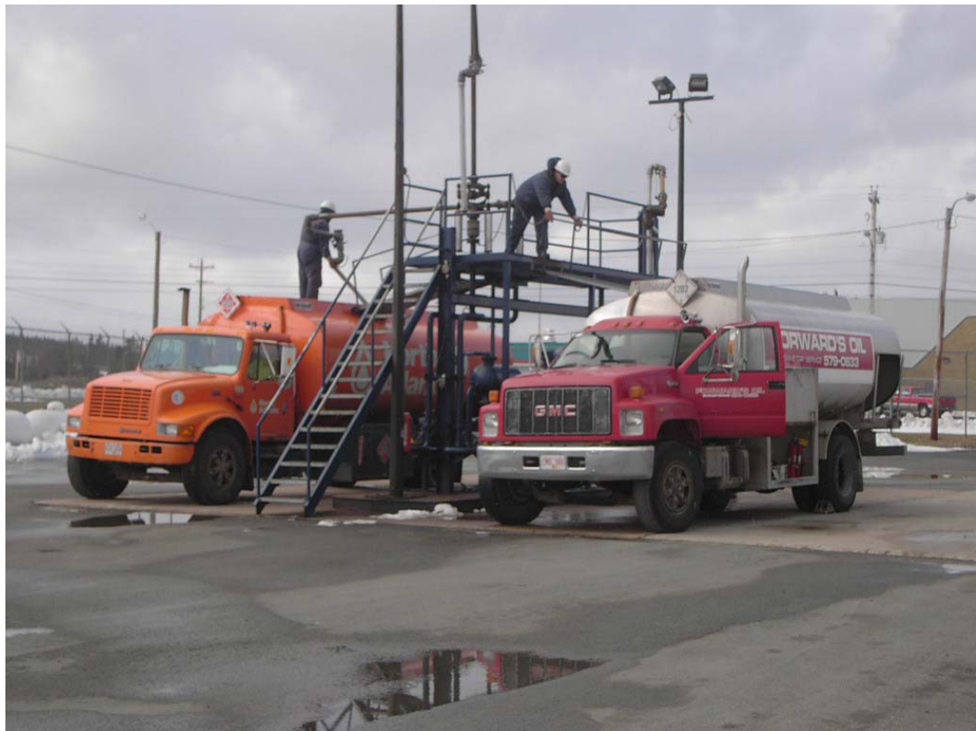
North Atlantic Bulk Plant – Loading Rack - Donovans – Mount Pearl
