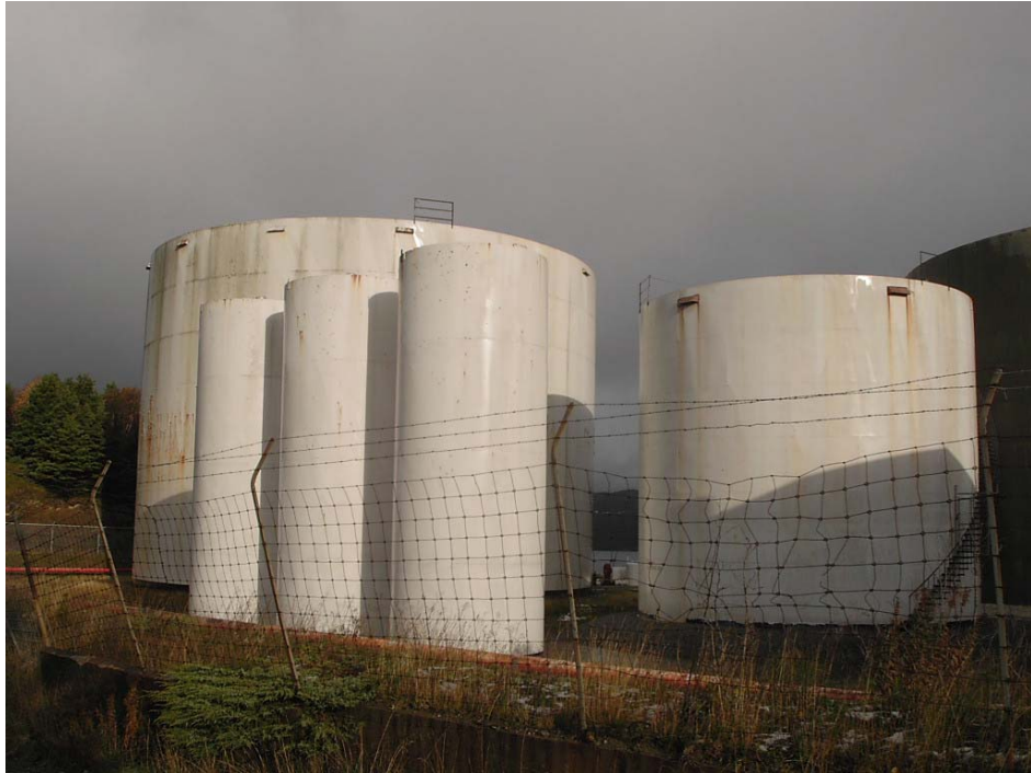
Irving Oil – Marine Terminal – Corner Brook – Being Decommissioned
