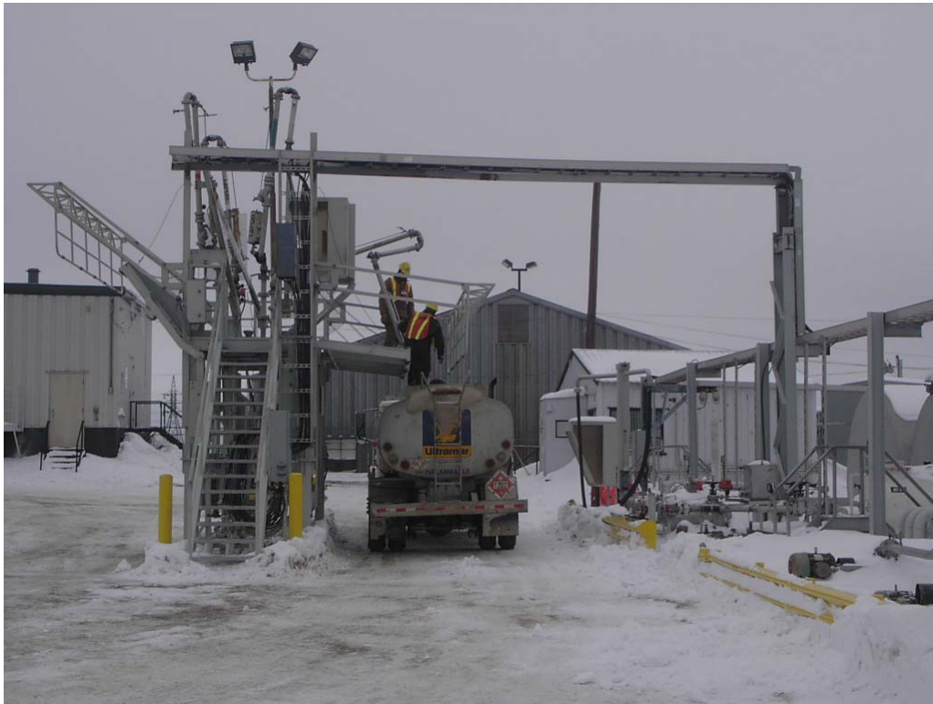
Rail Car Bulk Plant – Labrador City
