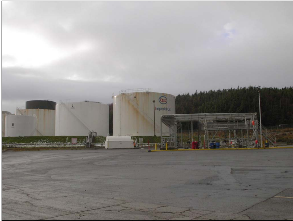
Imperial Oil – Primary Marine Terminal – Corner Brook
