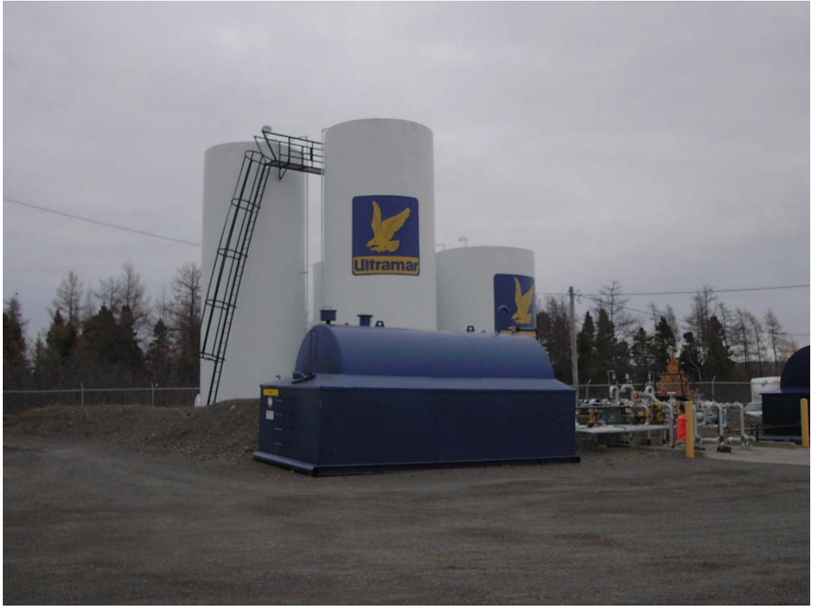
Ultramar - Bulk Plant – Lewisporte – Reportedly Being Decommissioned
