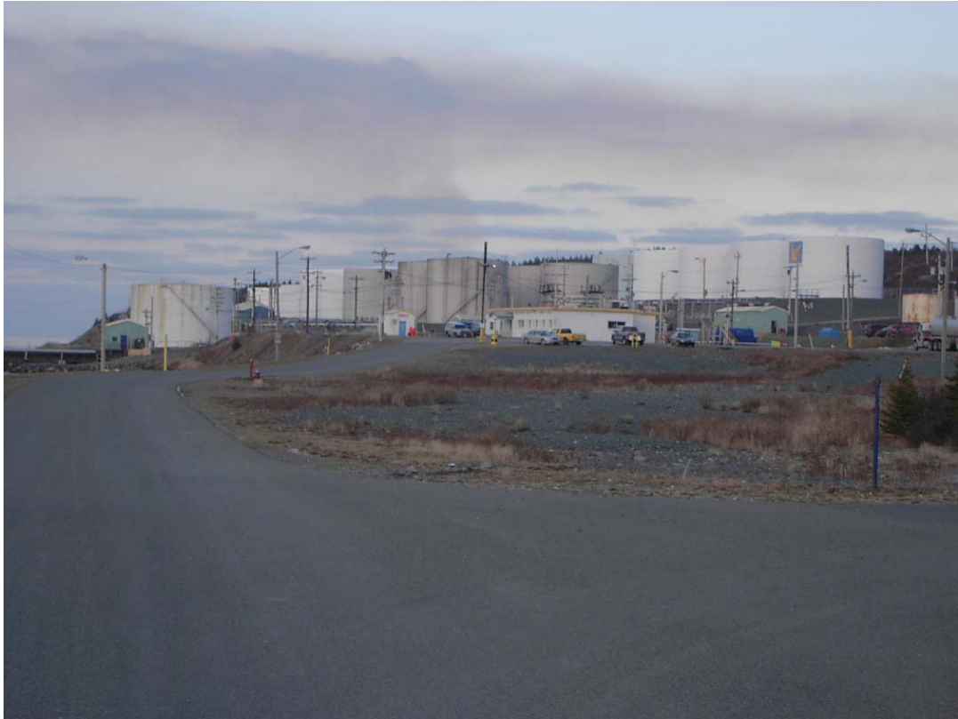
Ultramar Primary Marine Terminal – Holyrood
