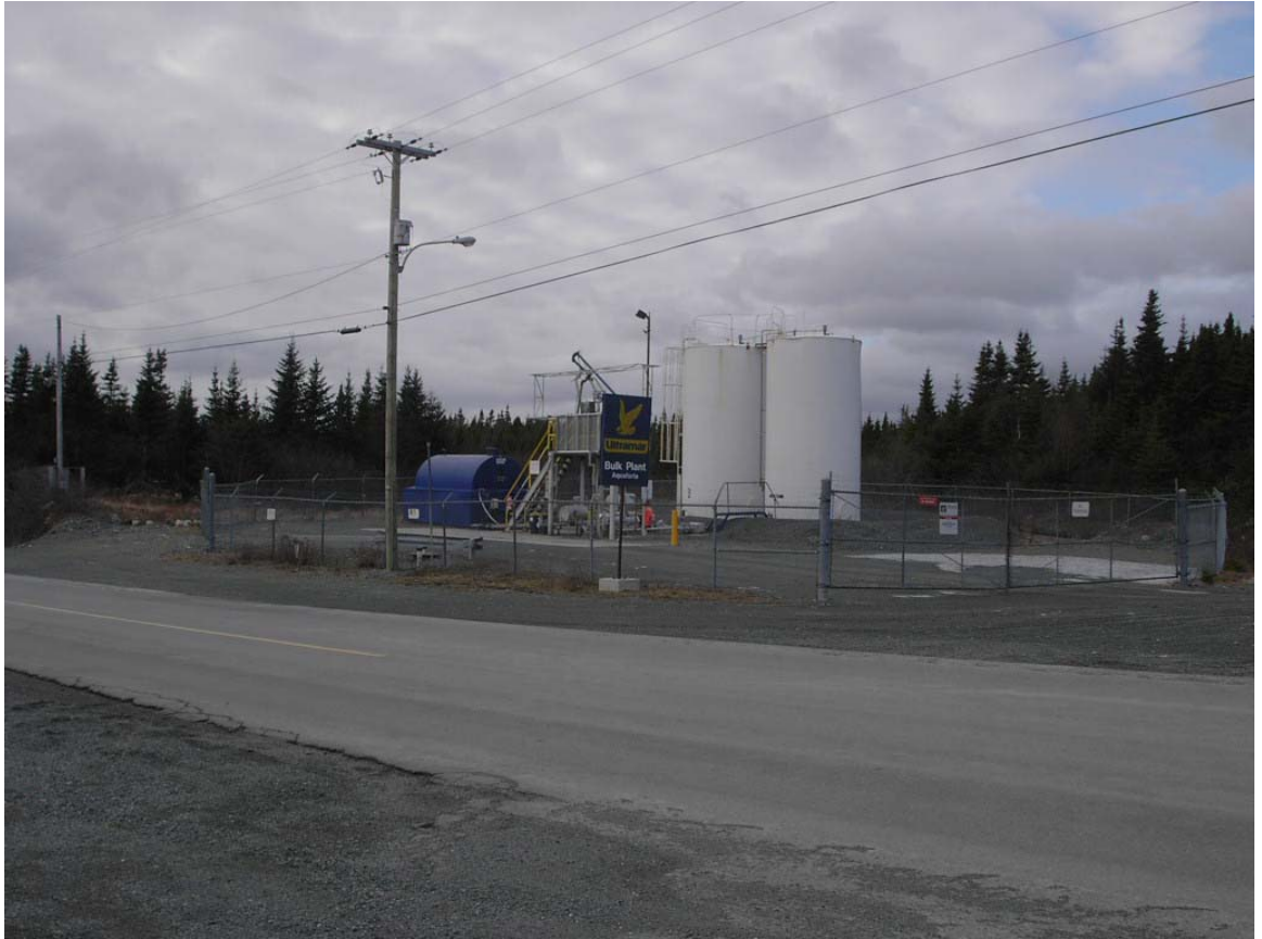
Ultramar - Home Heat Bulk Plant – Aquaforte
