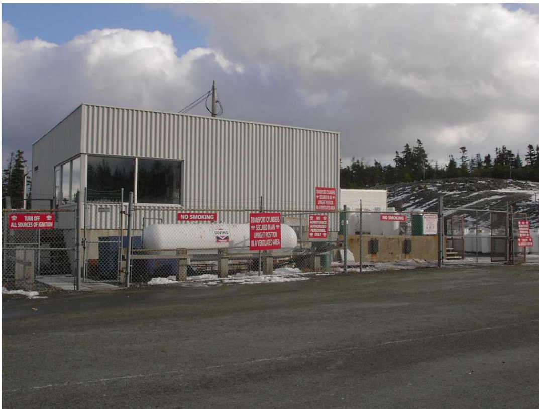
Irving – Propane Storage Plant - Donovans
