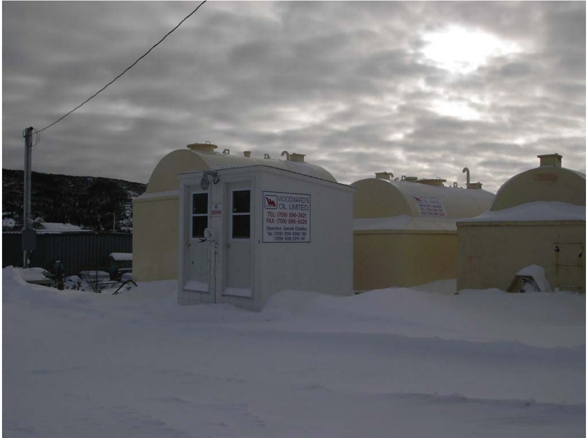
Woodward – Marine Depot – St. Lewis
