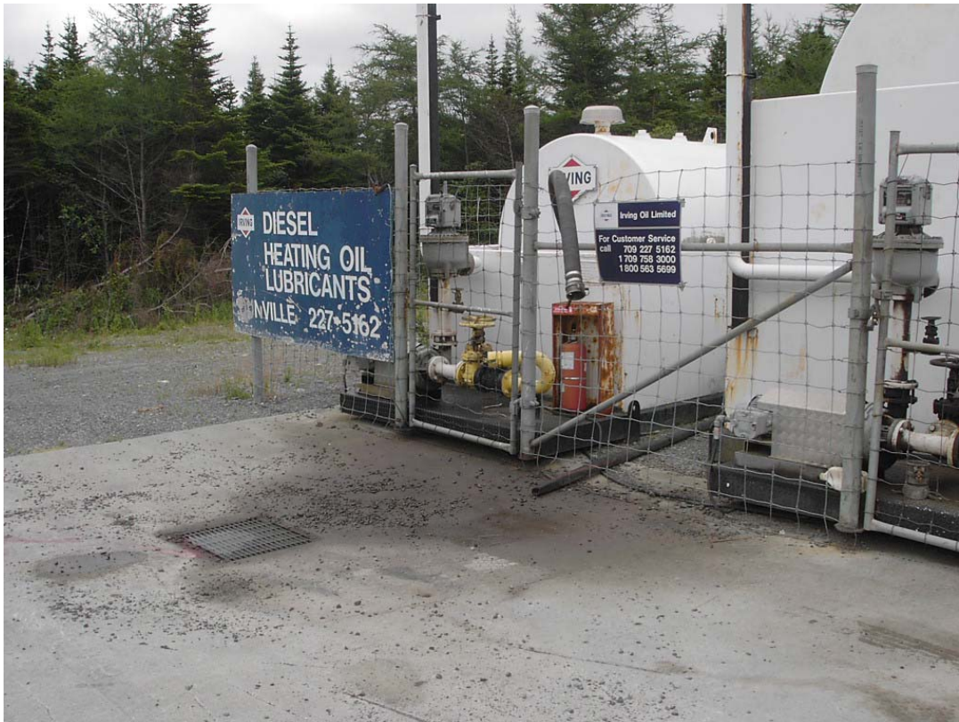
Irving Oil – Distillate Bulk Plant – Dunville - Reportedly Decommissioned
