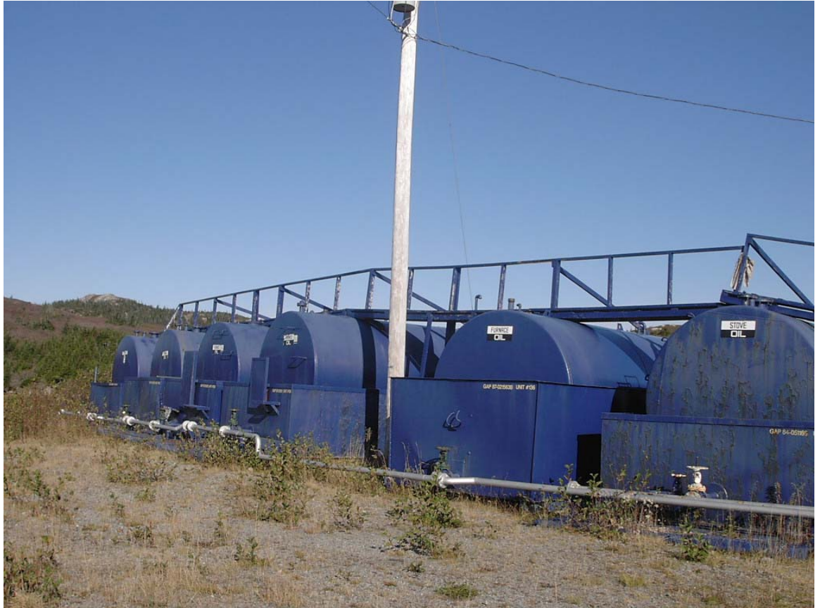
Former Western Petroleum – Bulk Plant – Burgeo – Being Decommissioned
