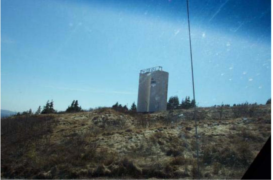
Irving Oil – Decommissioned Bulk Plant Tanks – Bell Island
