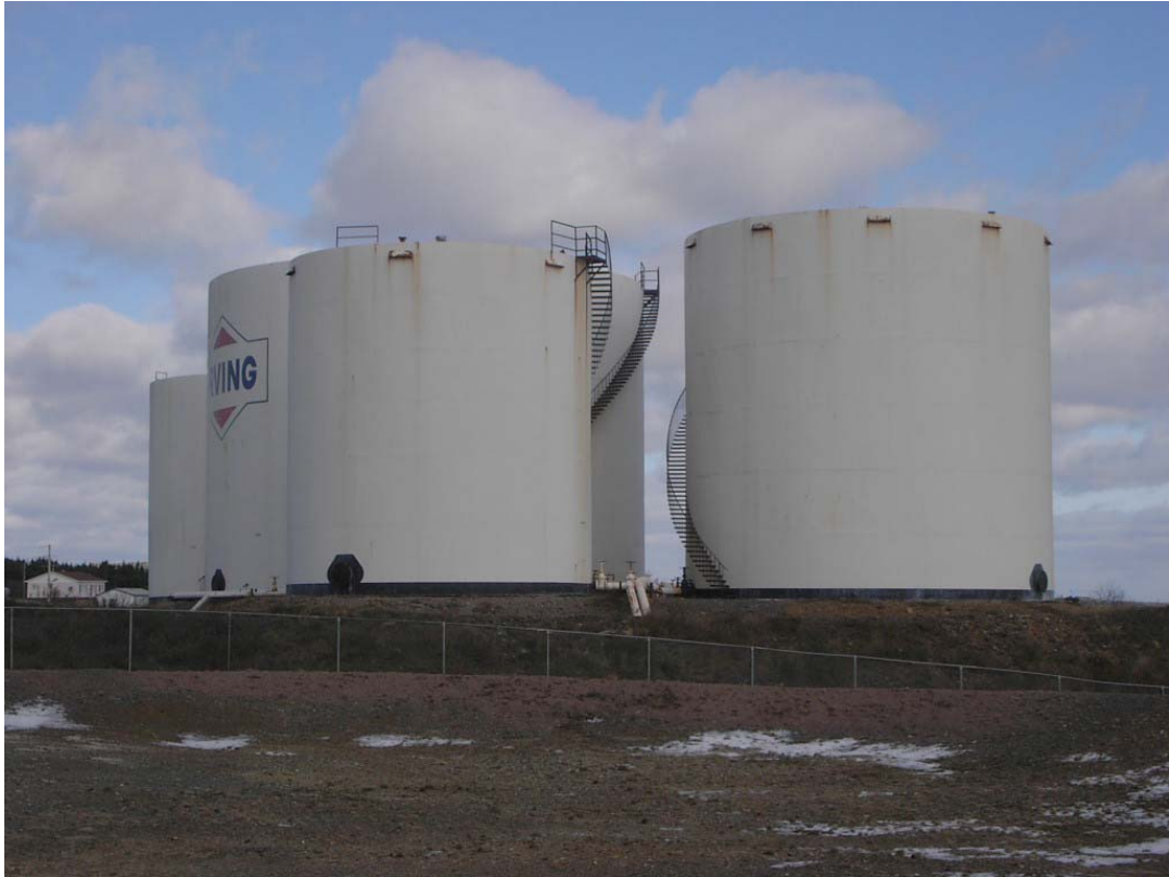
Irving – Secondary Marine Terminal – Marystown - Reportedly Decommissioned
