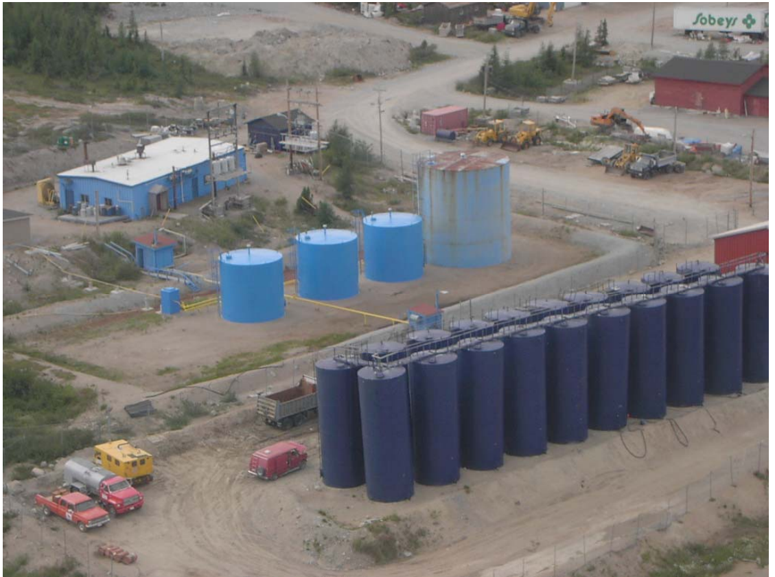
Woodward – Marine Depot – Nain (Newfoundland and Labrador Hydro tankage in background)
