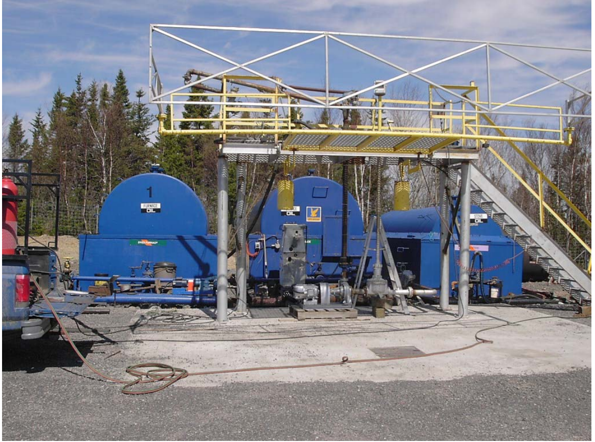
New Bulk Plant –R &B Services (Eli Russell) -Lethbridge
