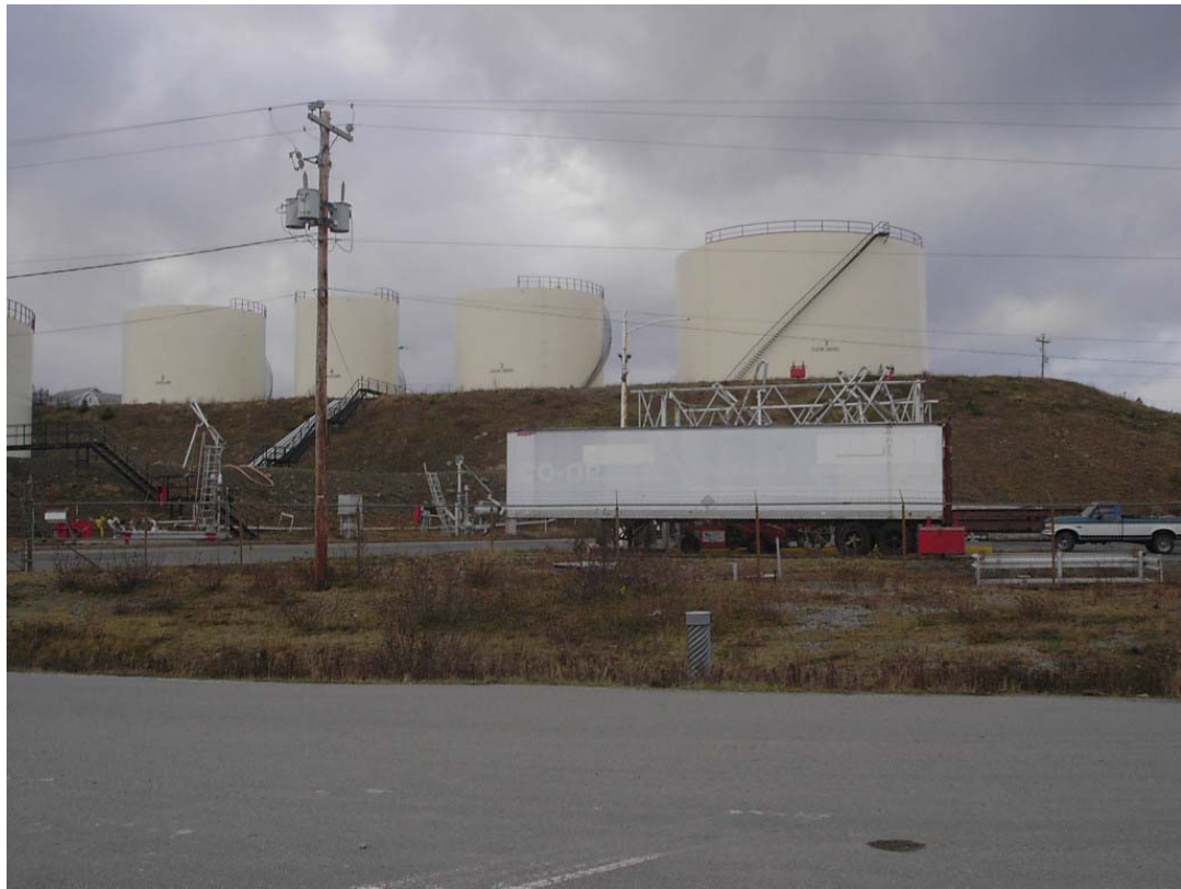
Woodward's Oil – Marine Terminal – Long Pond
