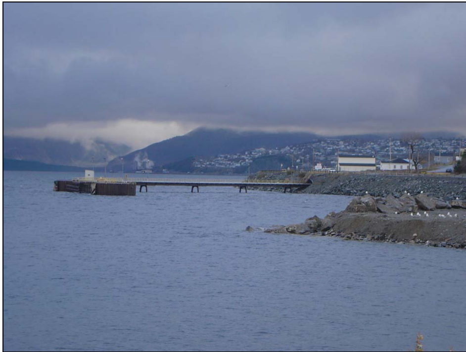
Ultramar – Primary Marine Terminal – Dock
