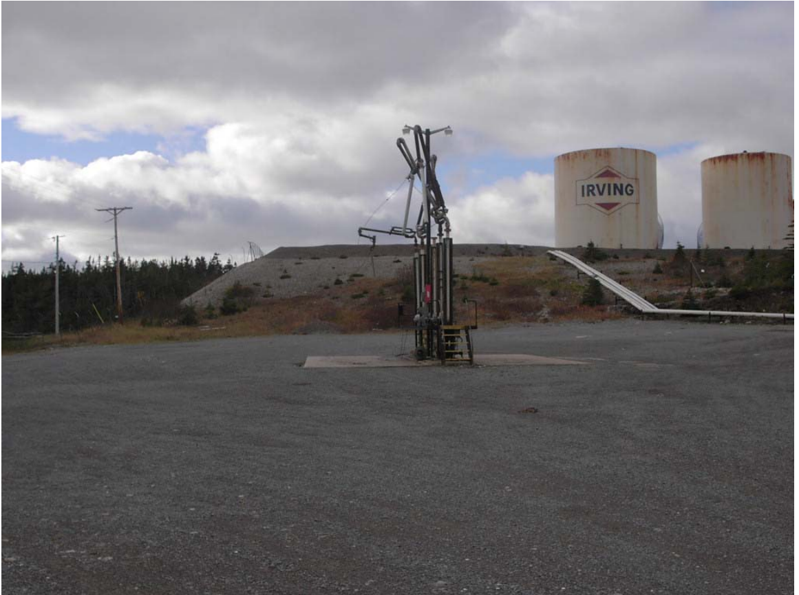
Irving – Bulk Plant – Port au Choix - Decommissioned
