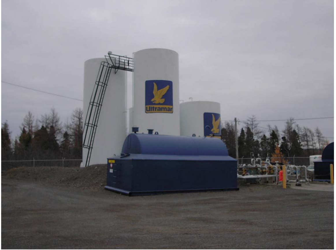
Ultramar - Bulk Plant – Lewisporte – Reportedly Being Decommissioned
