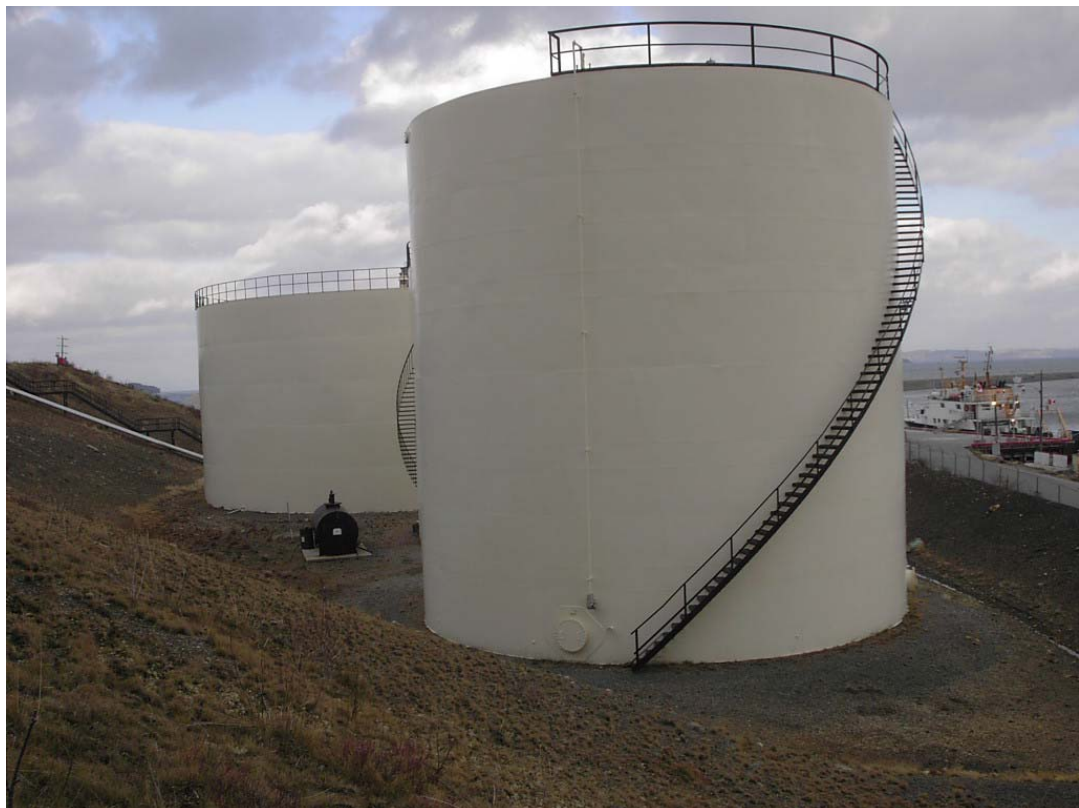
Woodward's Oil – Marine Terminal – Long Pond – Dock in Background
