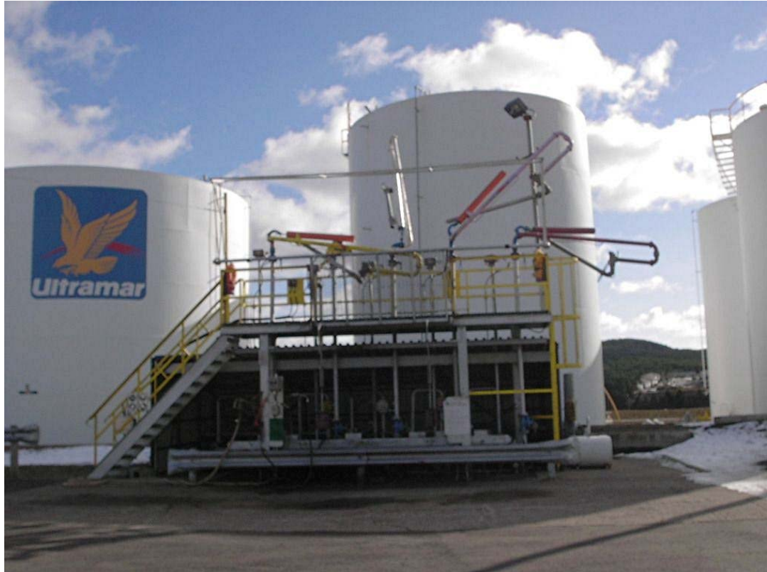
Ultramar – Secondary Marine Terminal - Marystown
