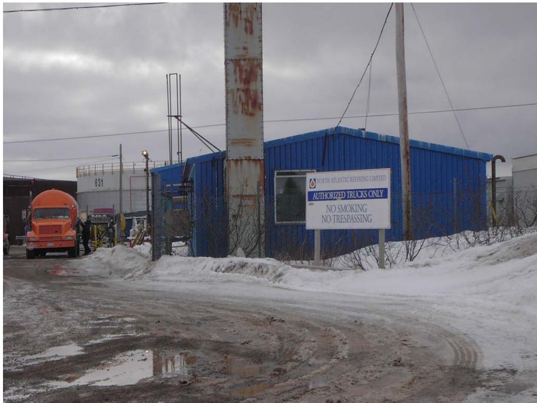
North Atlantic Refinery – Come By Chance – Loading Rack Area
