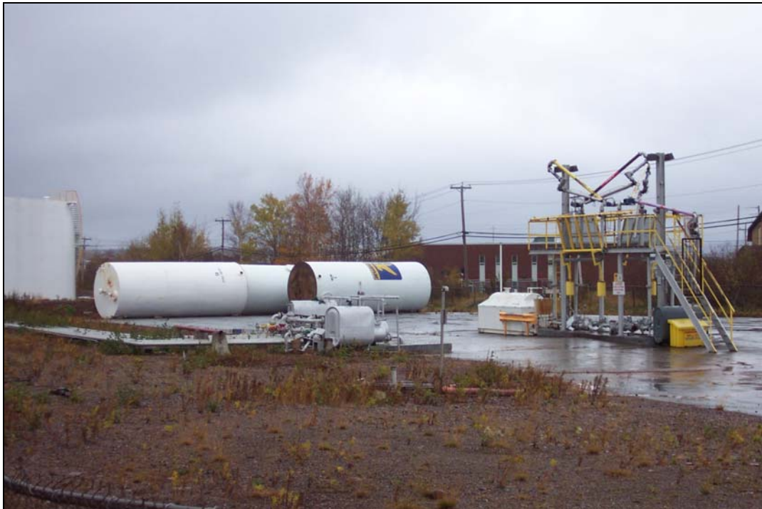
Ultramar – Marine Terminal – Botwood (Decommissioned and being dismantled)
