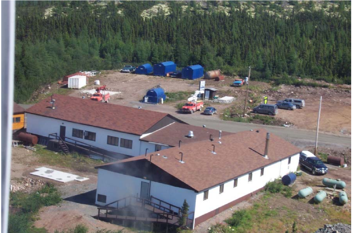
Normore – Decommissioned tankage from Marine Depot - Cartwright
