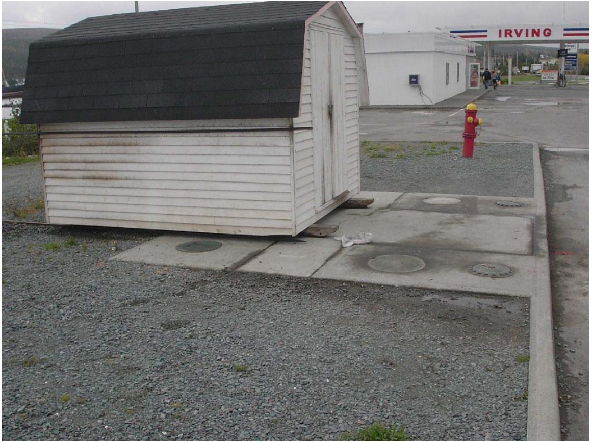
Irving Oil – Drop-Off Underground Heating Fuel Storage – Harbour Grace
