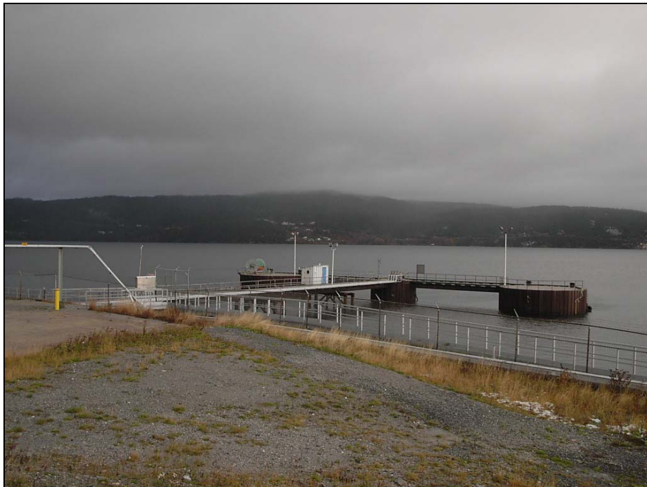
Imperial Oil – Primary Marine Terminal - Corner Brook - Dock
