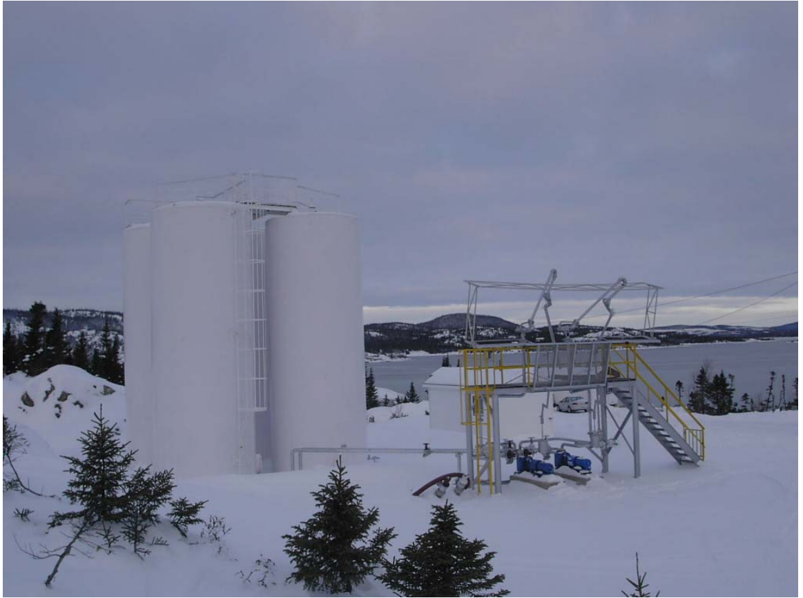
Normore – New Bulk Plant – Charlottetown – Labrador (Gasoline and Heating Fuel Storage)
